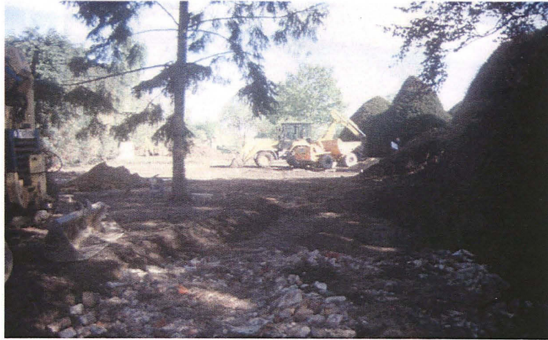
Plate 1 - General view of the site, looking north
