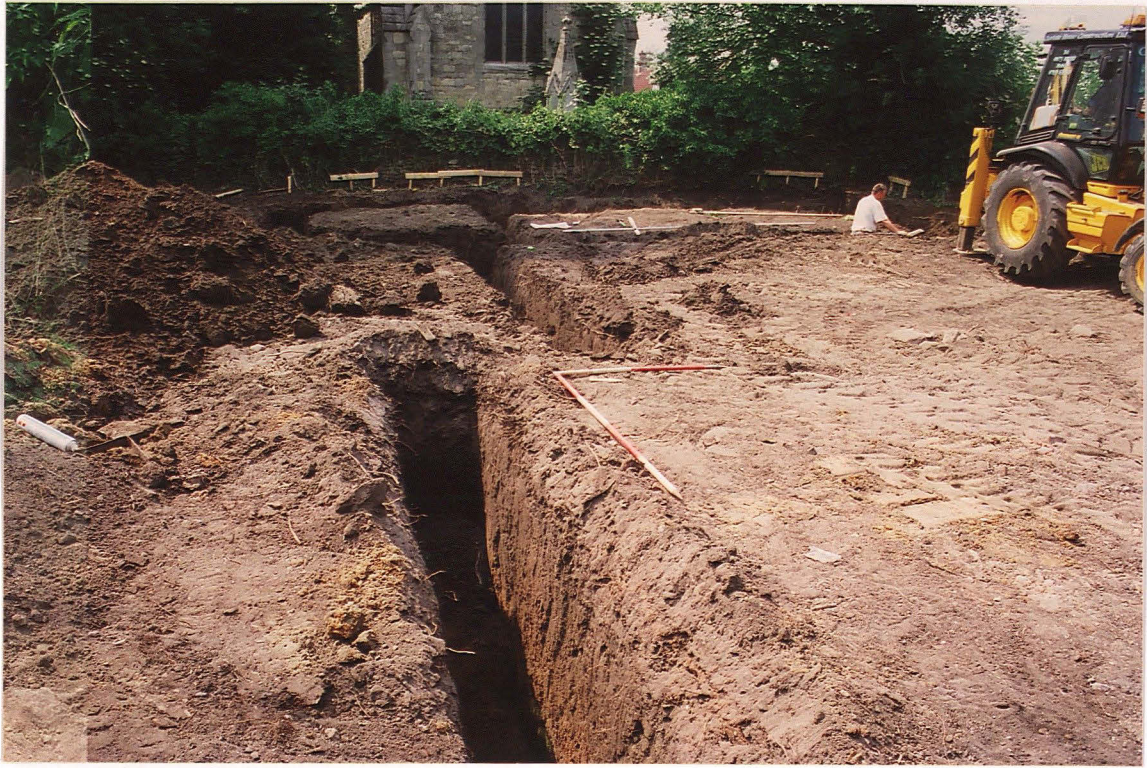
Pl. 2 Foundation trench for back wall of house.
