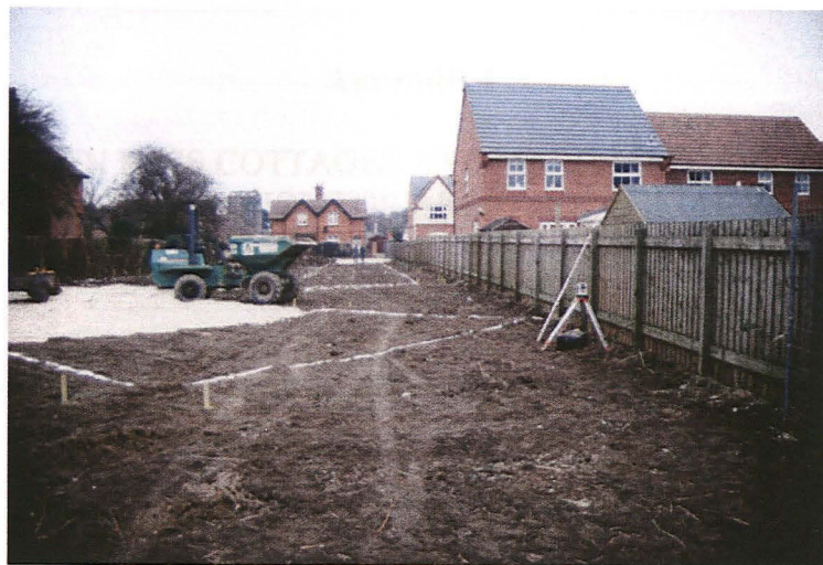
Plate 1 - General view of the site, looking north
