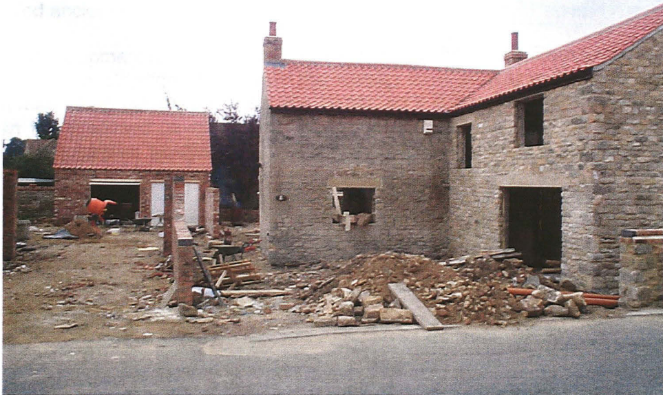
Plate 2 View of site, looking south.
