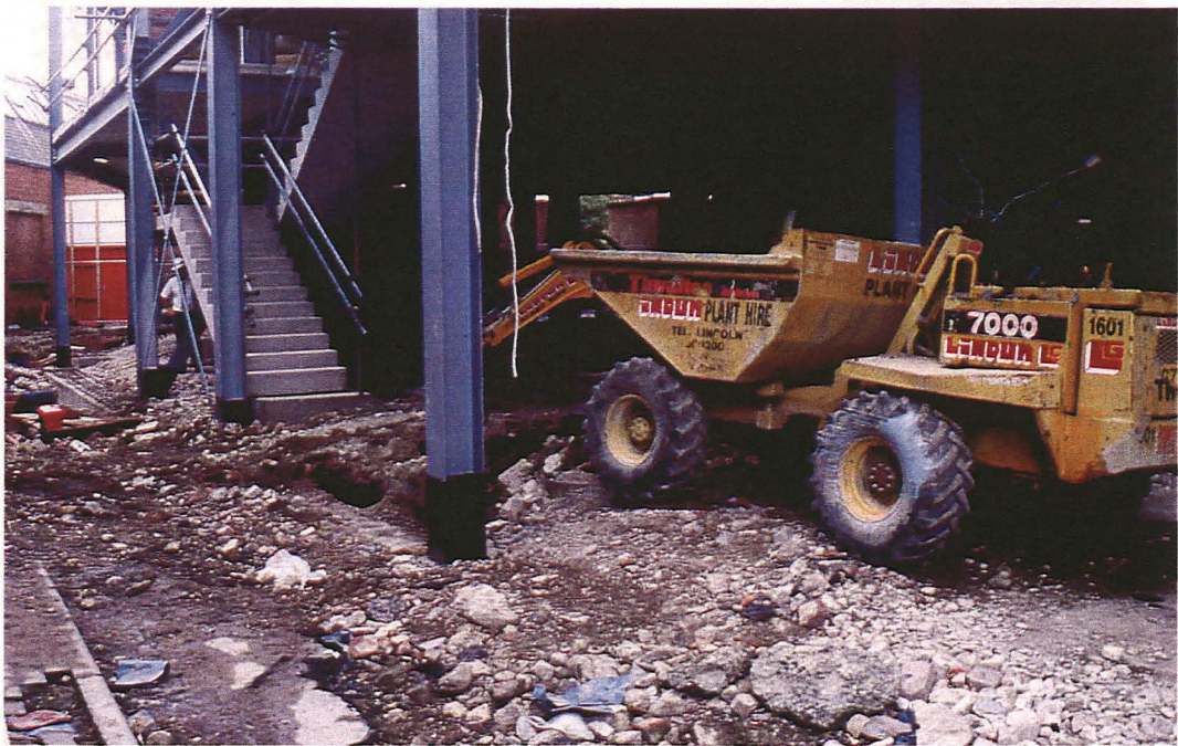
Plate 2 Area of lift shaft, prior to excavation, looking west
