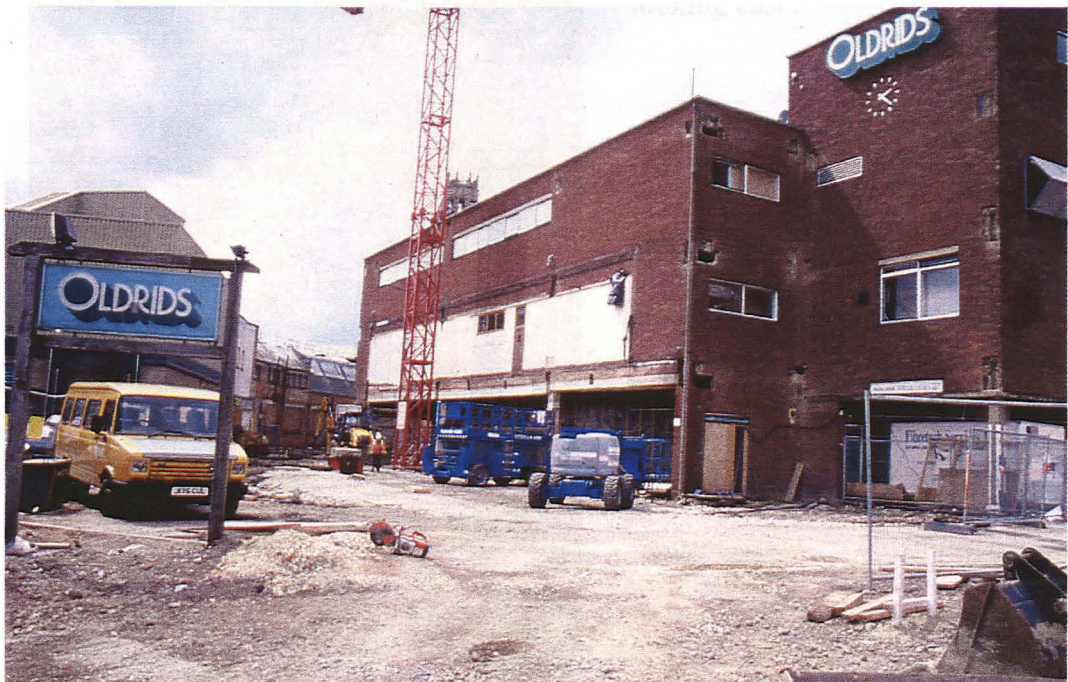
Plate 1 View of entire site, prior to groundworks, looking northwest
