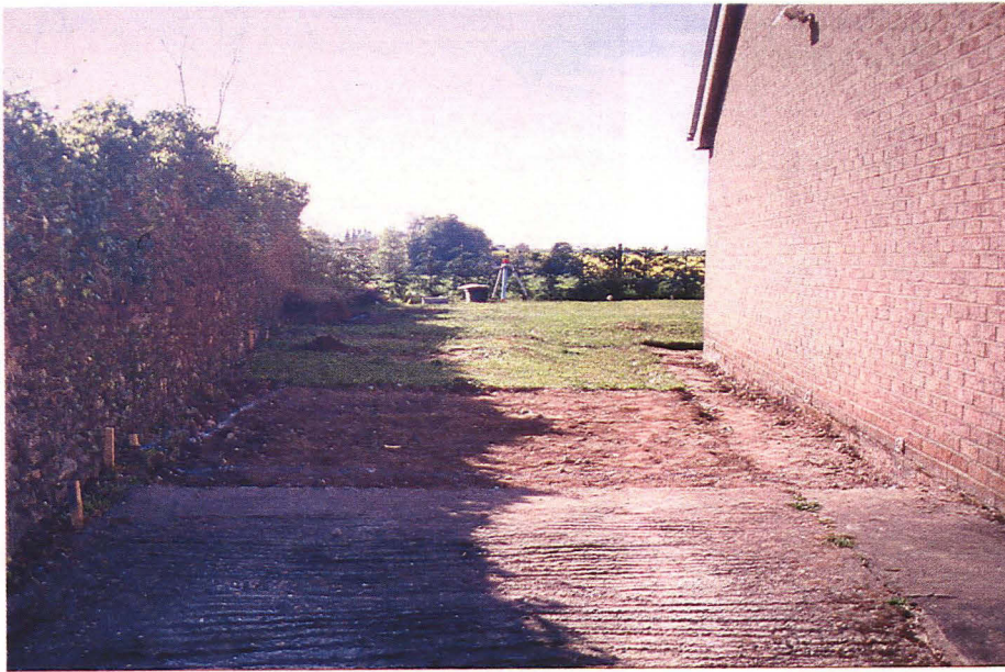
Plate 1 General view of site prior to groundworks looking south
