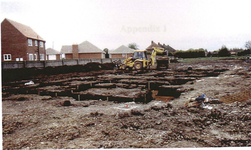
Plate 9 Plot 2, General view foundation trenches, looking southeast
