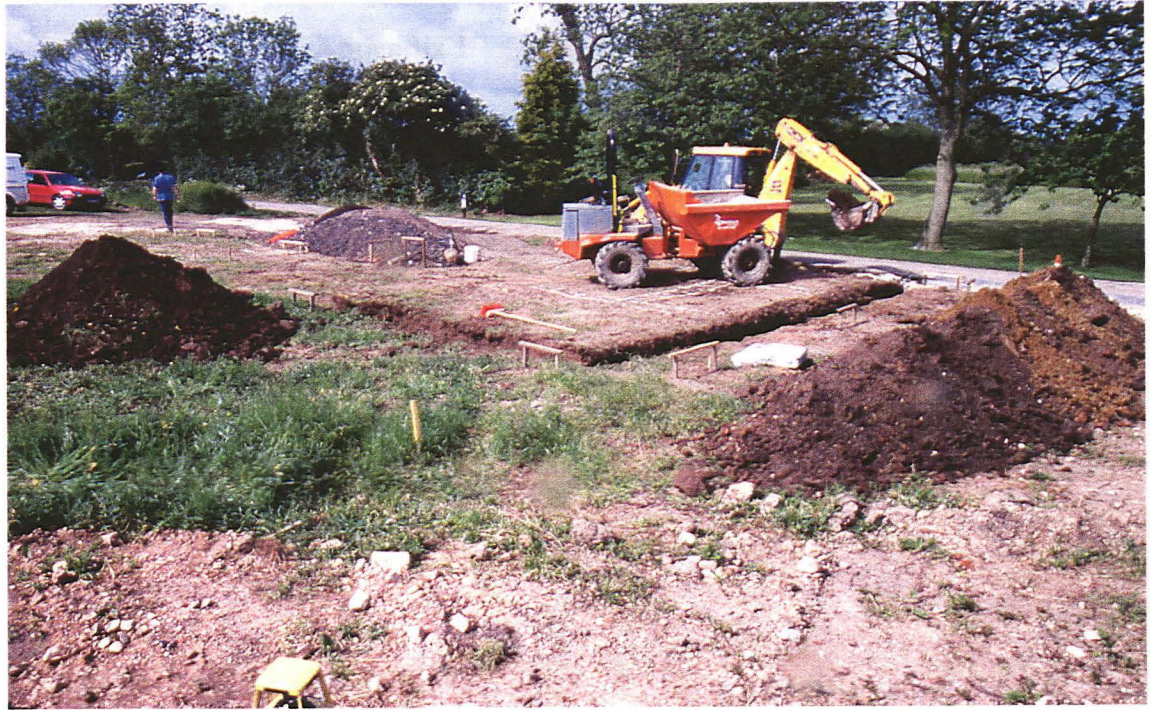
Plate 1 General view of site at commencement of groundworks looking west
