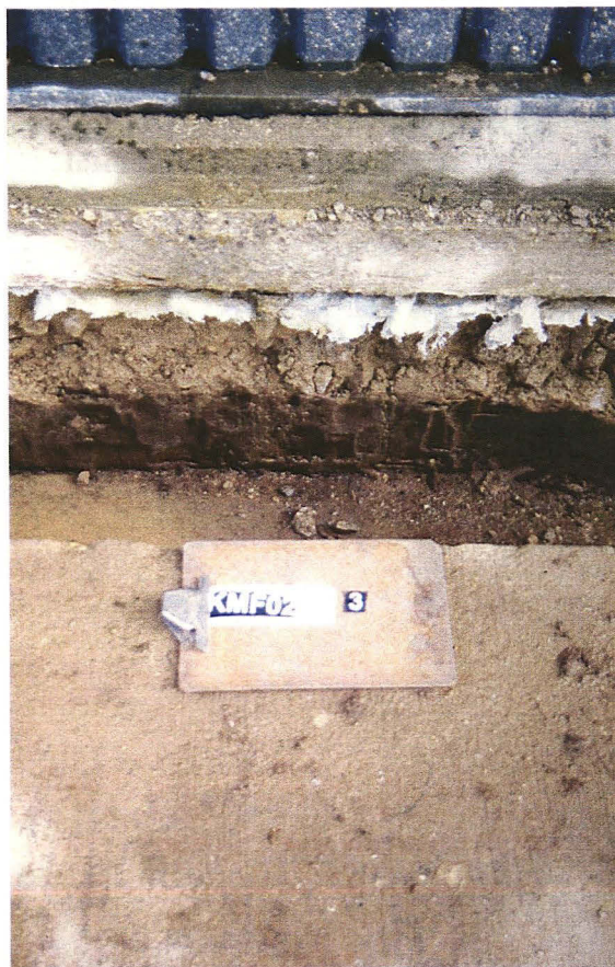
Plate 2 Section 1, looking north
