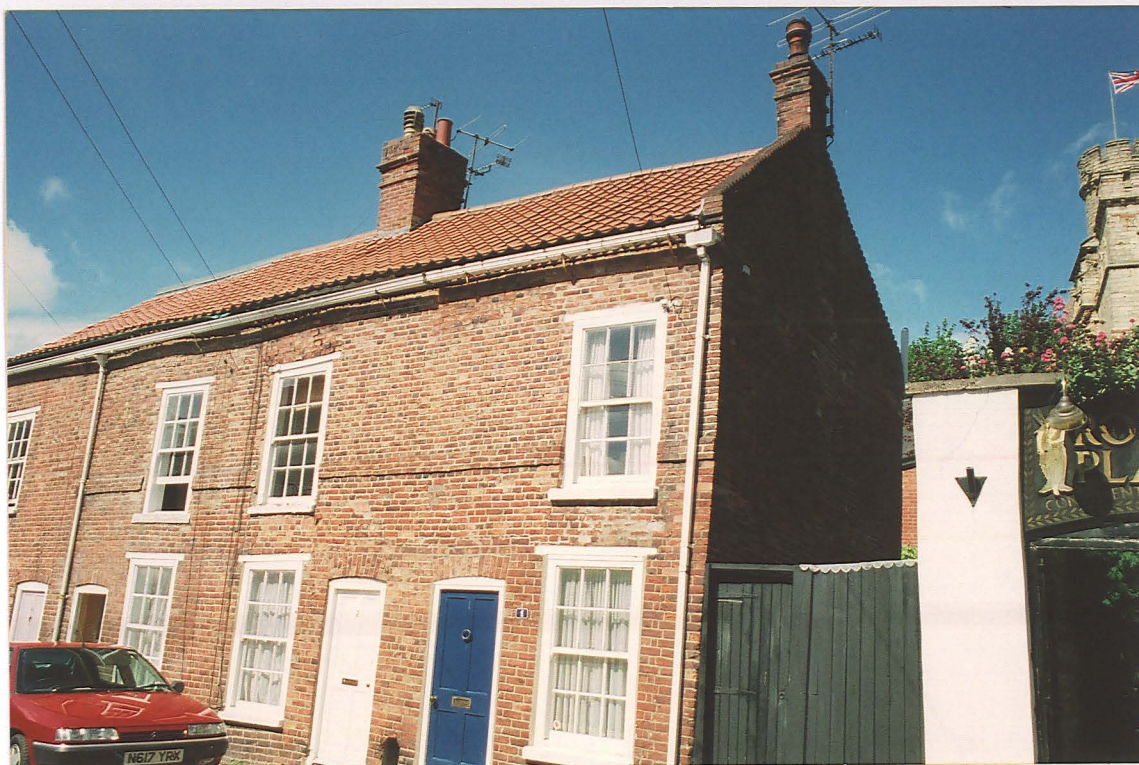
Pl. 1 Drury Lane, front elevation of Nos. 1-3 showing string course marking original eaves height, with earlier roofline on gable end.
