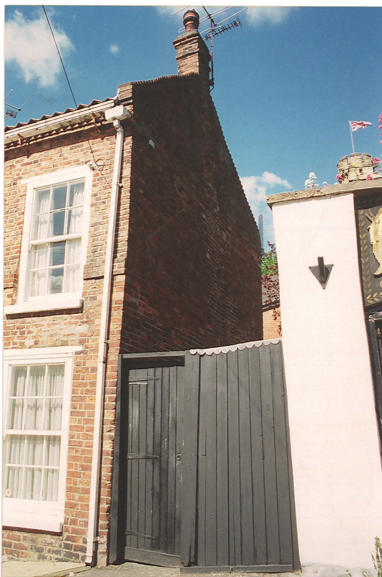
Pl. 2 Close-up view of north gable end showing earlier roofline and chimney.
