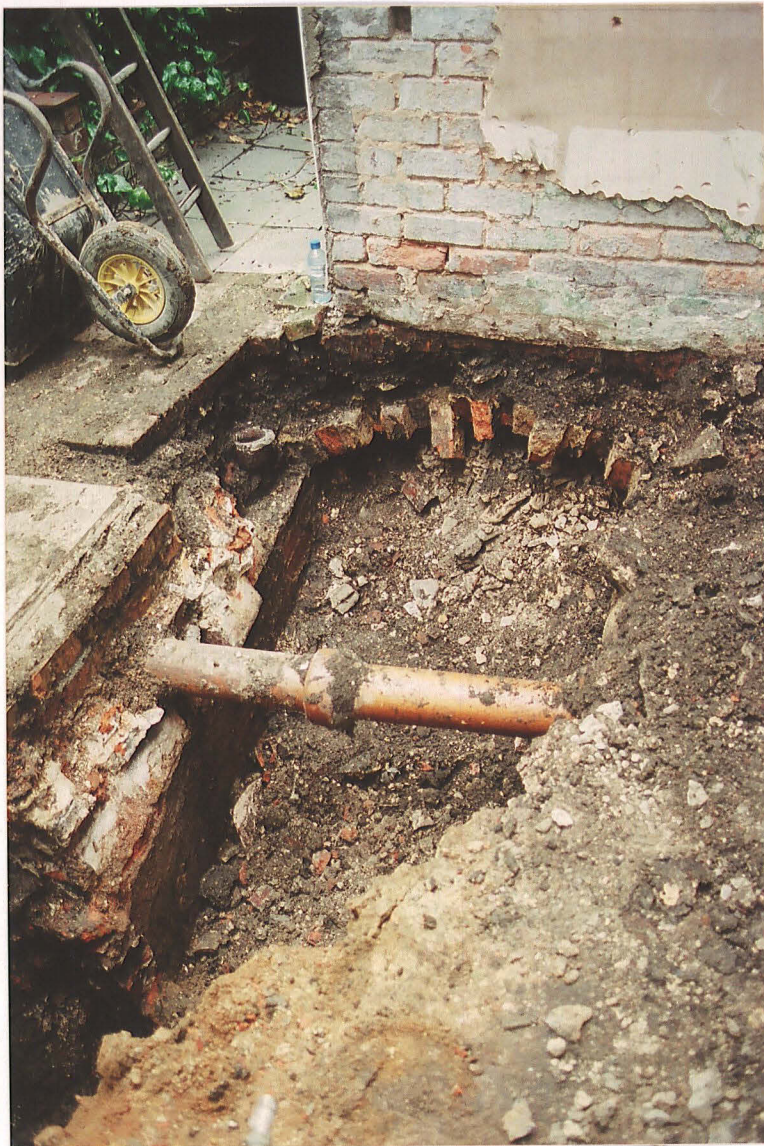
Pl. 5 Cellar after vaulting has been removed, running beneath adjacent extension to No. 2 (top) with soil pipe and inspection chamber resting on cellar wall (left) looking NW.
