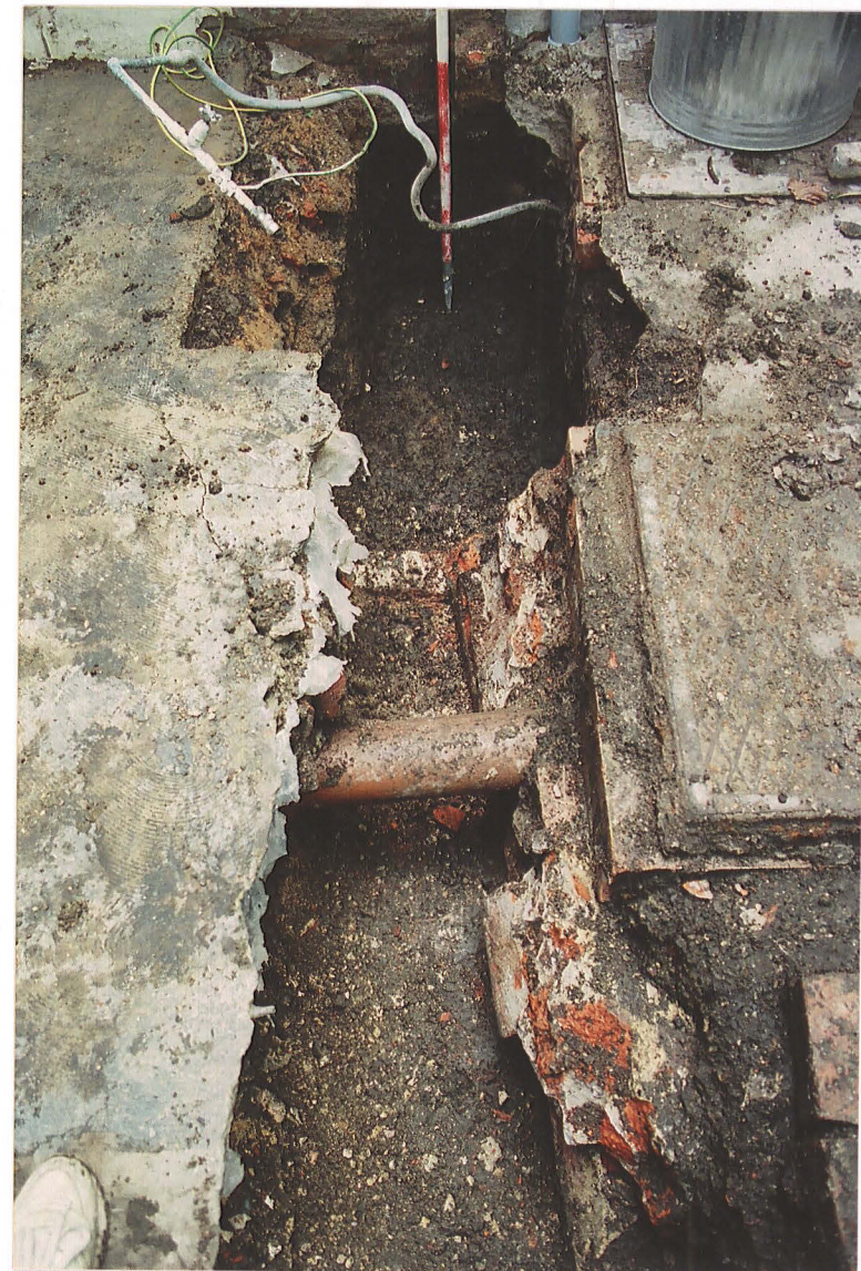
Pl. 7 Close-up of cellar vault showing earlier soil pipe 104 capped with an earthenware lid.
