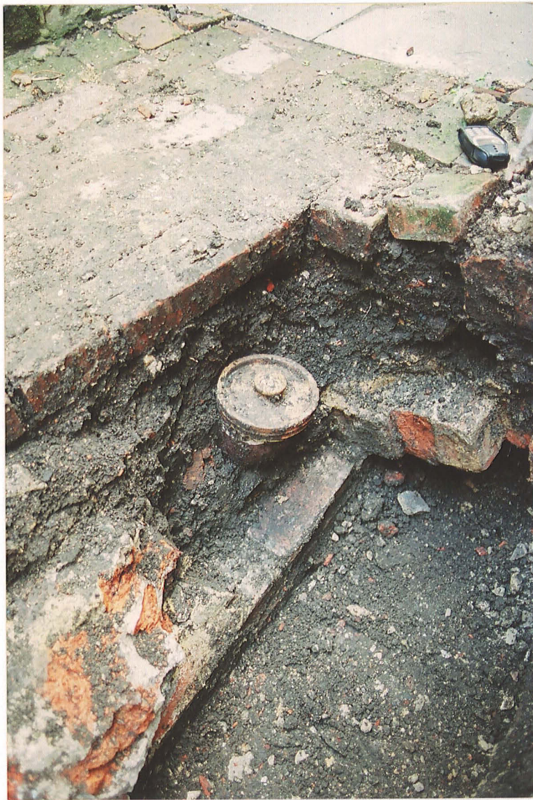
Pl. 7 Close-up of cellar vault showing earlier soil pipe 104 capped with an earthenware lid.
