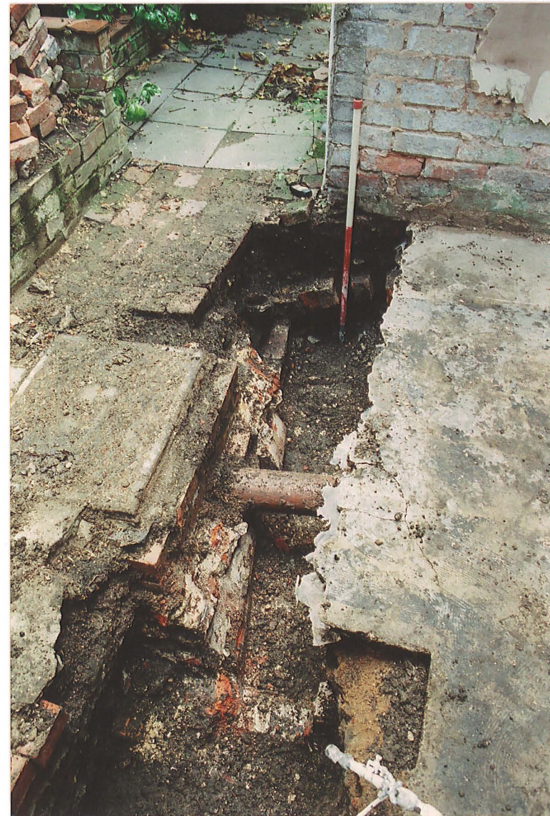
Pl. 5 Cellar after vaulting has been removed, running beneath adjacent extension to No. 2 (top) with soil pipe and inspection chamber resting on cellar wall (left) looking NW.
