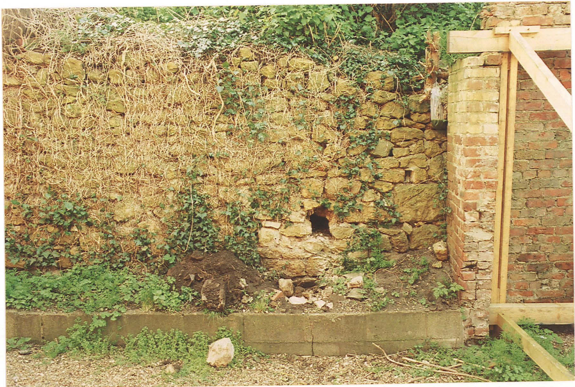
Pl. 9 Borehole 2 at the west end of the retaining wall.
