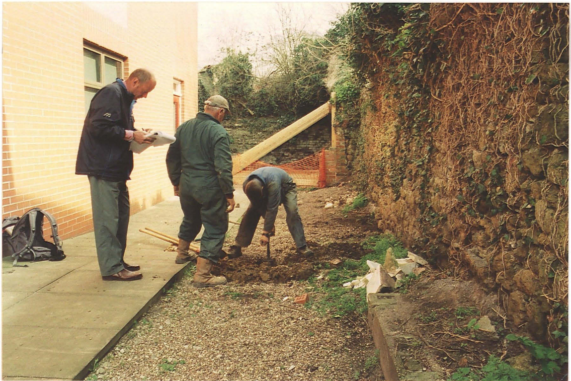
PI. 10 Test pit/auger hole on external side of the retaining wall.
