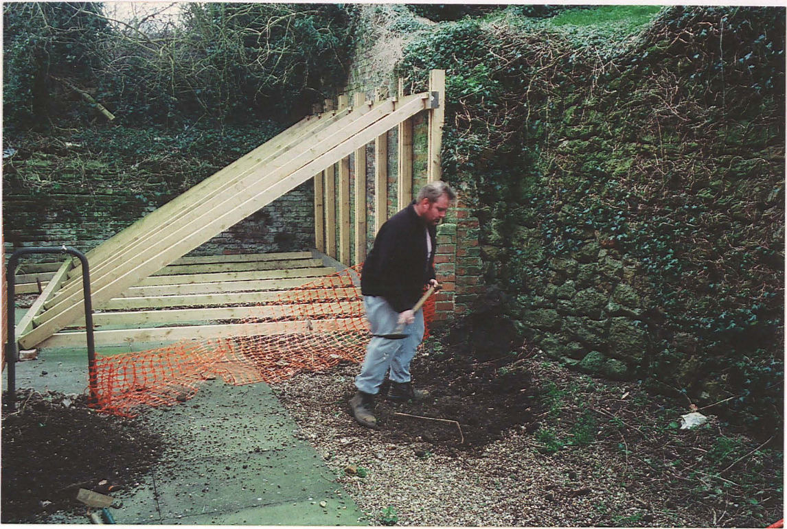
Pl. 1 Evaluation trench location during clearance.
