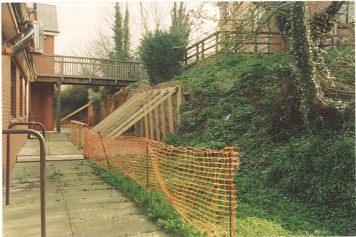
PI. 11 View of retaining wall and sloping ground beyond, looking north-east.
