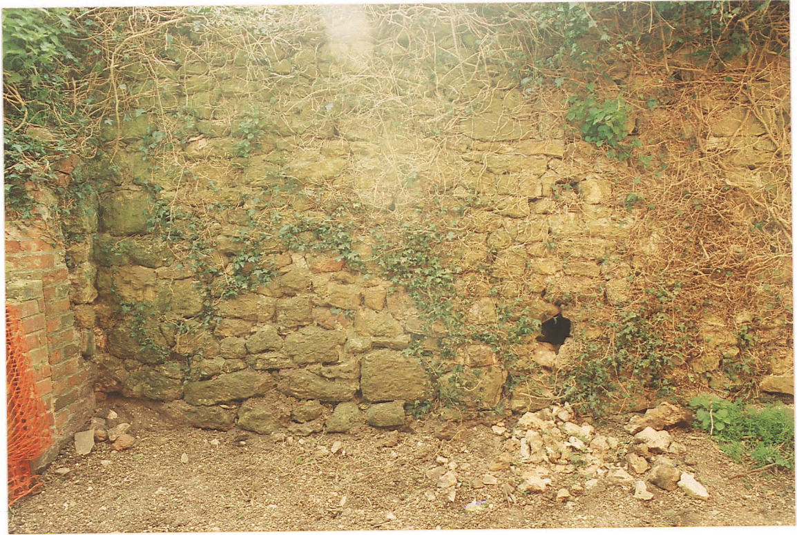
Pl. 8 Borehole 1 at the east end of the retaining wall.
