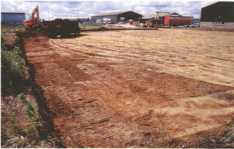
Plate 1 - General view of the development area during topsoil stripping, looking southwest
