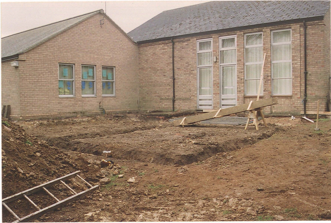
Pl. 2 Foundation trenches for the new extension (looking SE).
