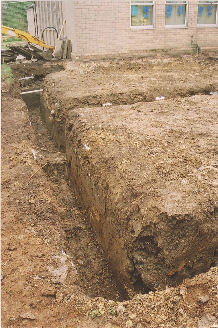
Pl. 4 Northern wall foundation trench, with the concrete backfill 22 visible at the northern end of the western return trench (looking NE).
