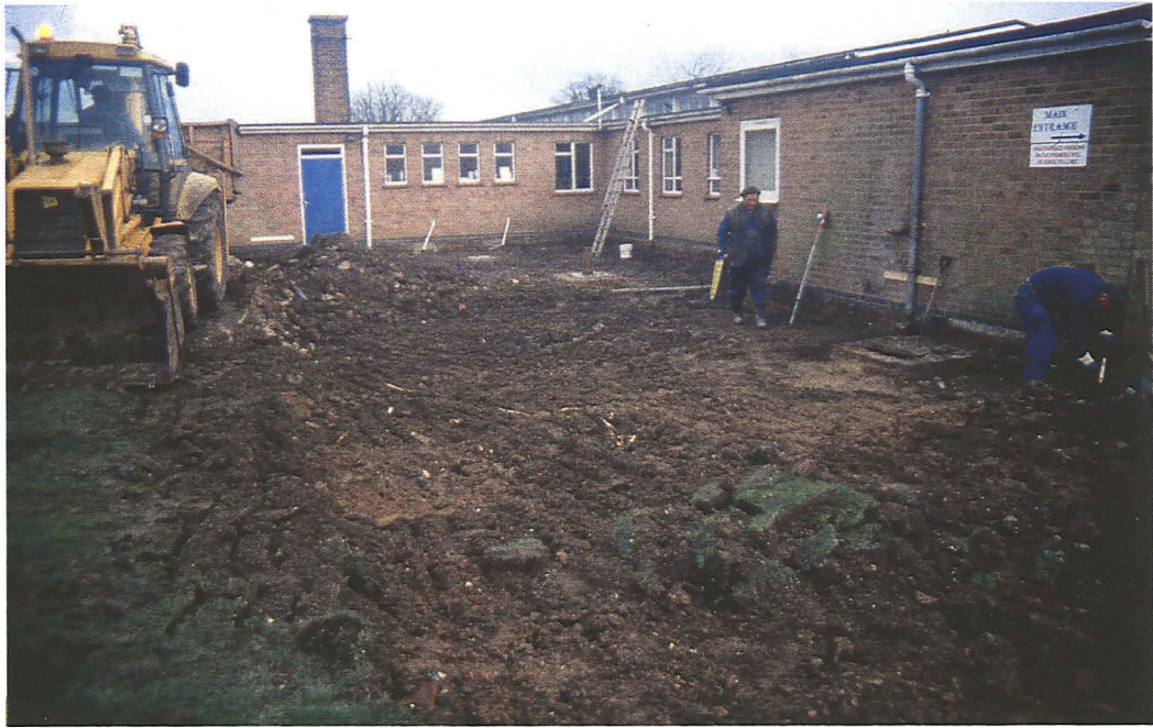
Plate 1 General view of stripped area looking east
