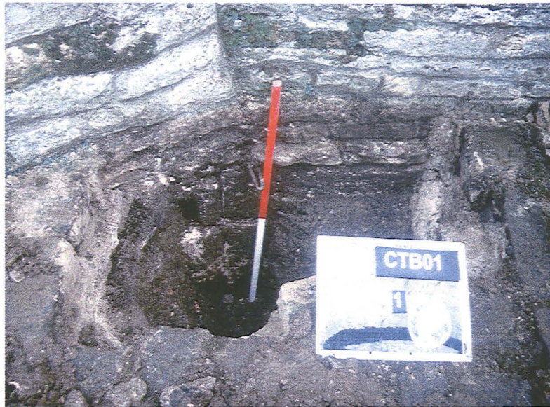
Plate 3 - Trial Pit 1, showing the exposed stonework, looking southeast
