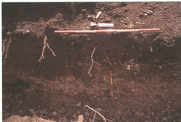
Pl.3: Shot of foundation trench, office extension, looking south-east
