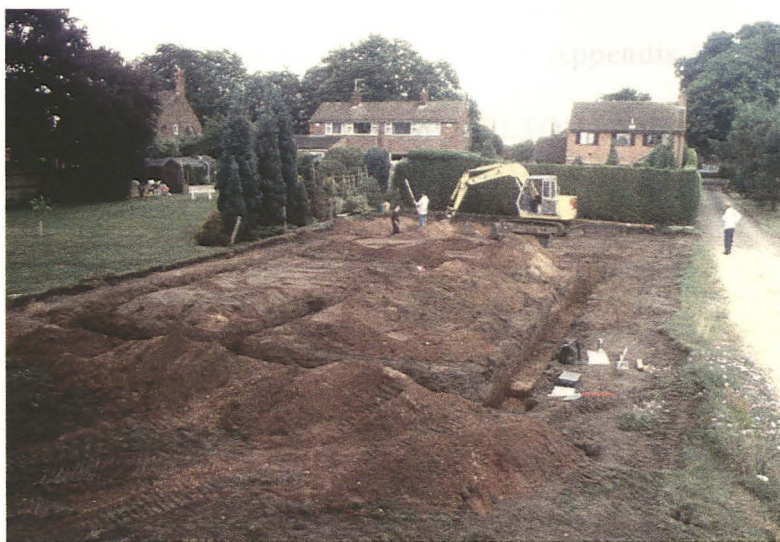
Plate 1 - General view of the site looking southeast towards Belton Lane
