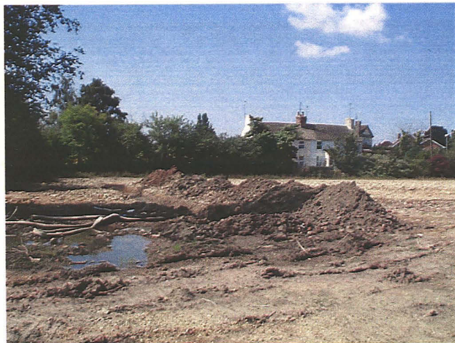
Plate 2 General view of Trench 10, looking southwest.
