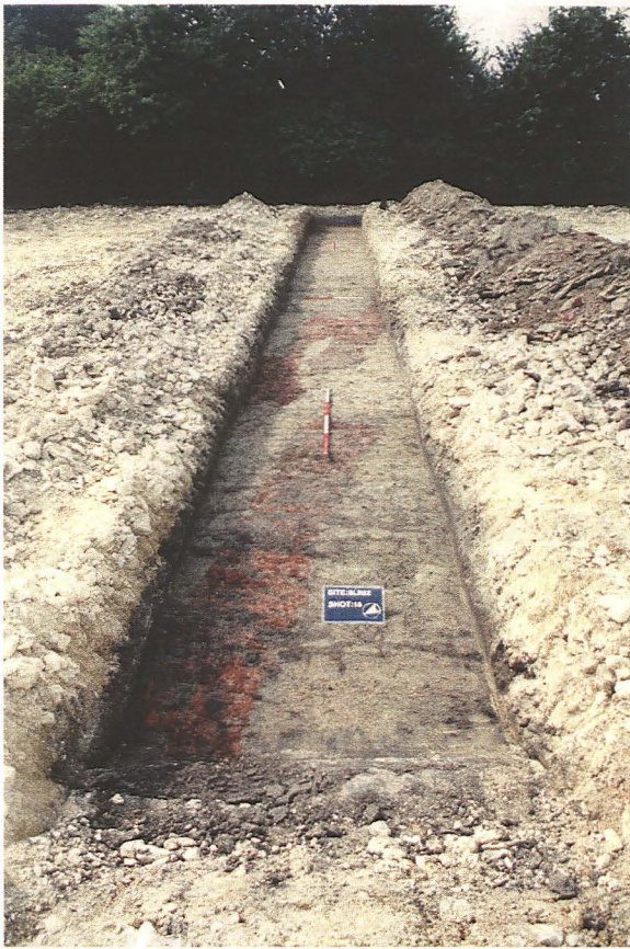
Plate 4 Trench 16 showing possible post-medieval brick clamp flues, looking southwest.
