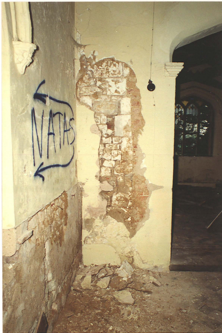
Pl. 28. North side of chancel arch showing brick facing of new arch.
