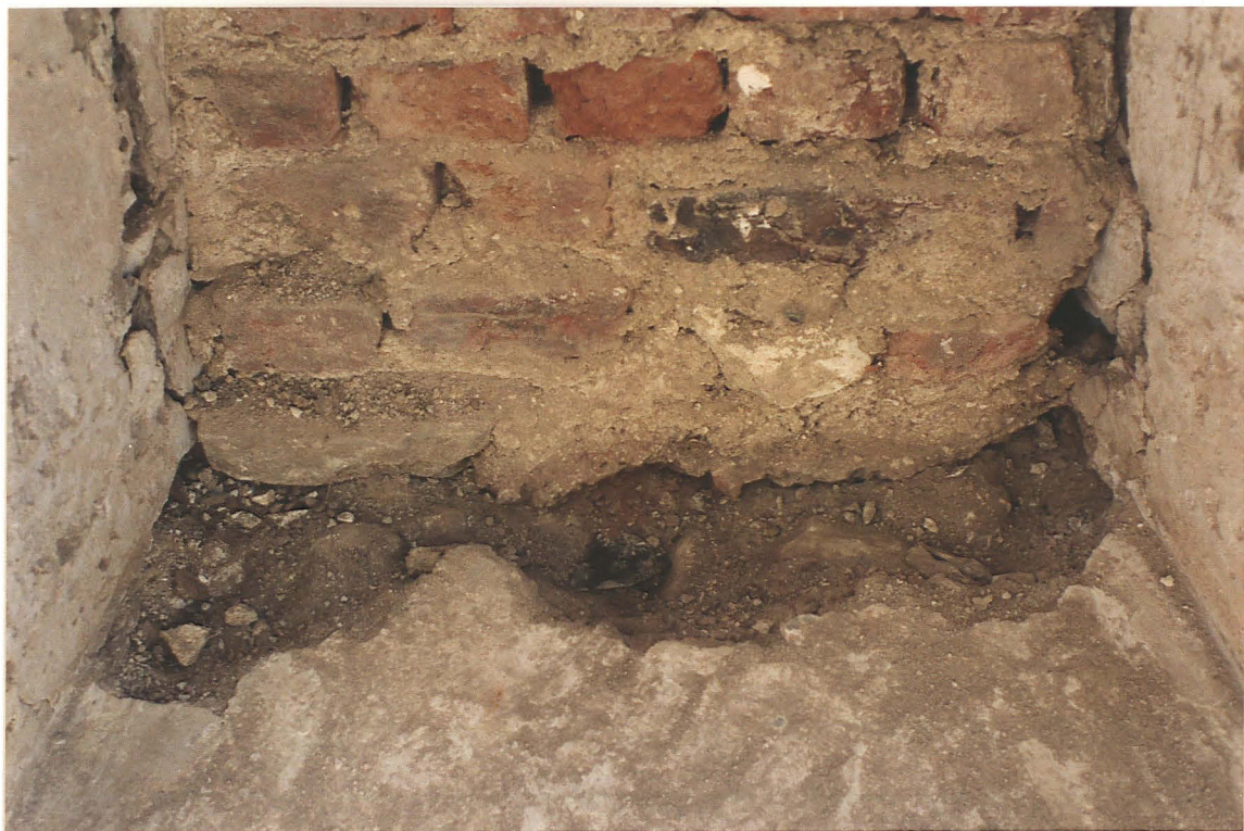
Pl.10. East window sill, showing glass in situ and external brick blocking.
