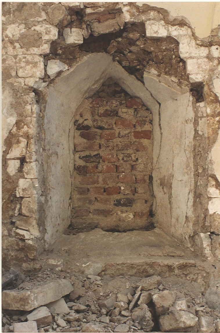
Pl.9. East window - after removal of brick blocking.
