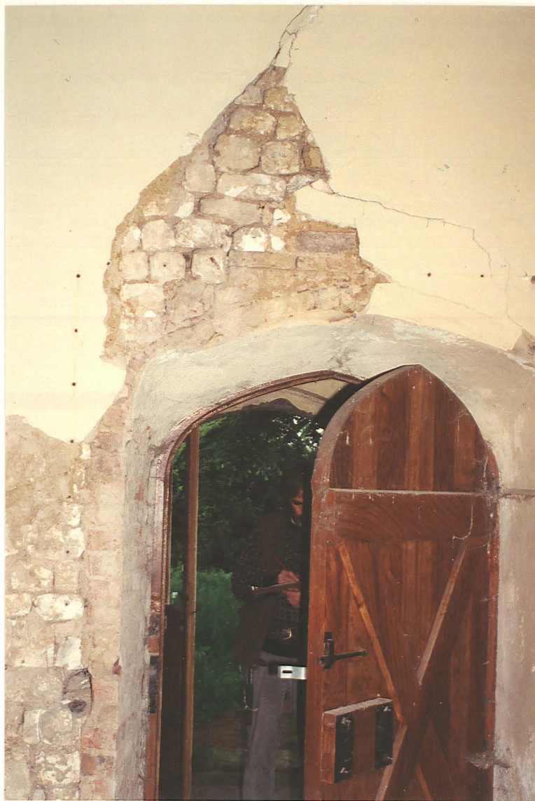
Pl.5. Entrance in south wall of nave.
