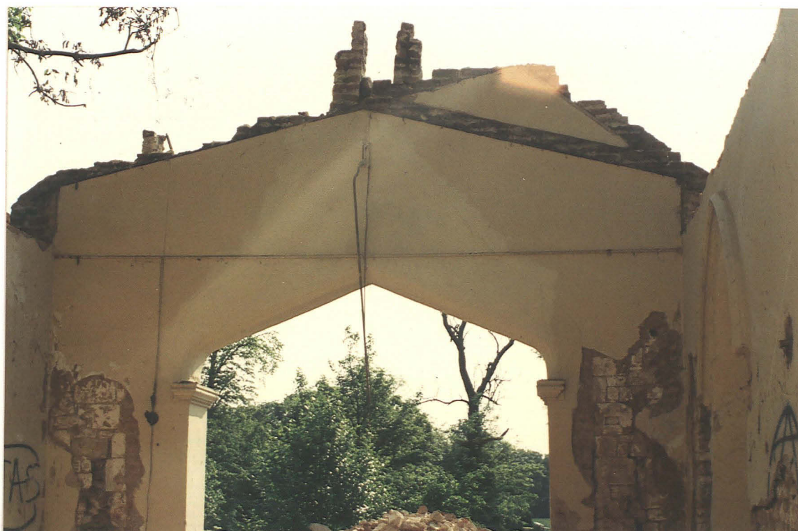
Pl. 26. Chancel arch looking towards chancel.
