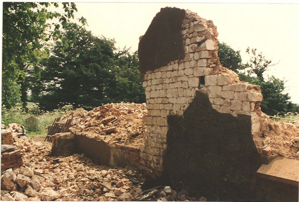
Pl.18. Nave north wall (exterior), showing chalk coursing, putlog hole and rubble core.
