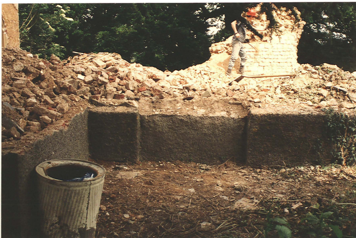
Pl.6. Nave south wall, (porch to left). Recess shows position of blocked doorway. Lower door pintle found on left side, just above demolition level.
