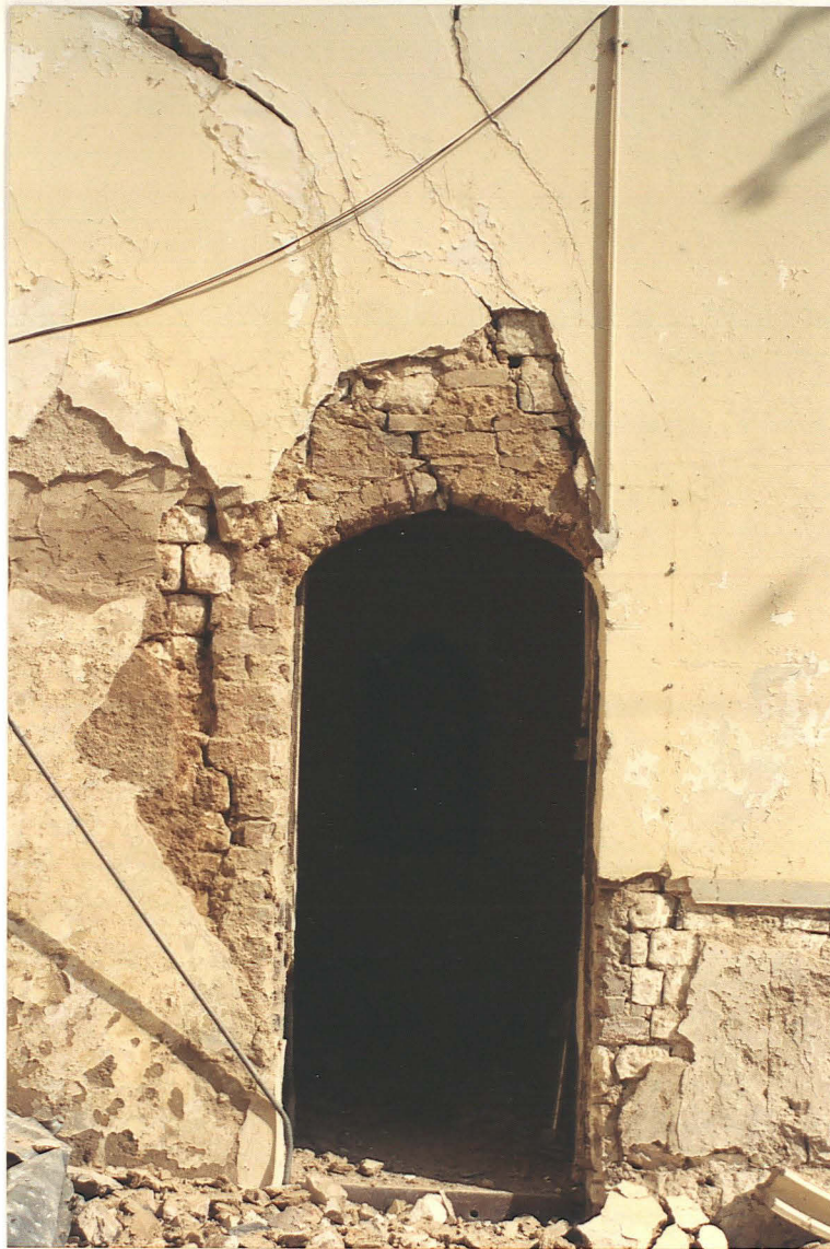
Pl.12. Nave north wall. Inserted vestry entrance.
