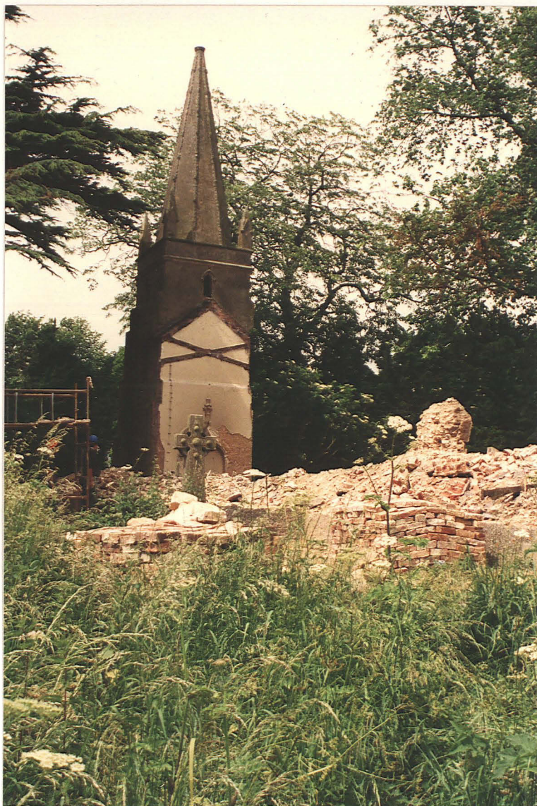
Pl.25. Free-standing brick tower after demolition of nave and chancel.
