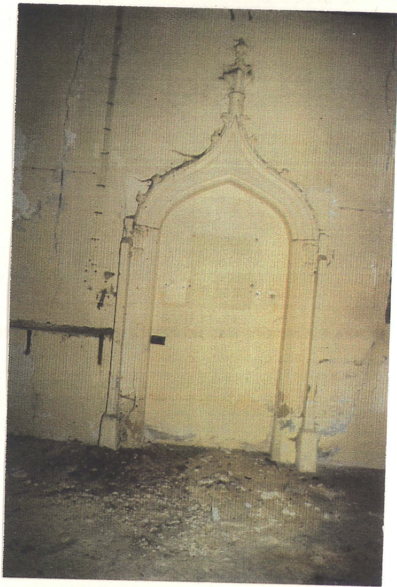
Pl.23. Tower arch, built 1837.
