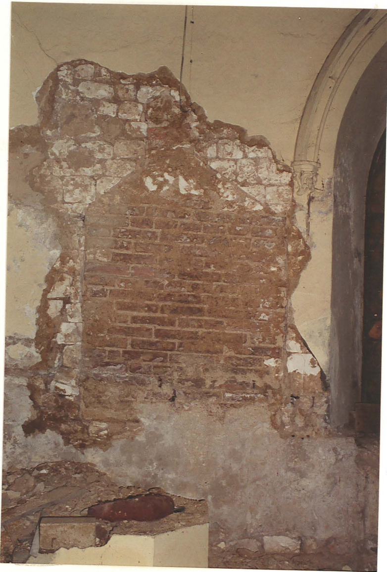
Pl.7. Blocked east window in south wall of nave.
