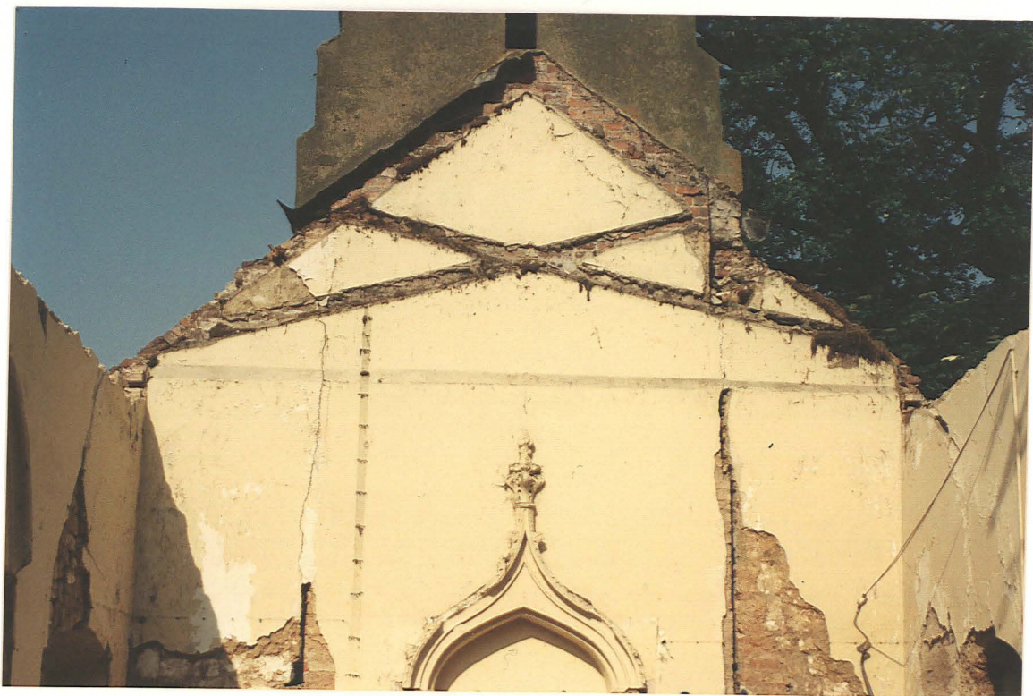
Pl.24. Inserted tower, vertical joint.
