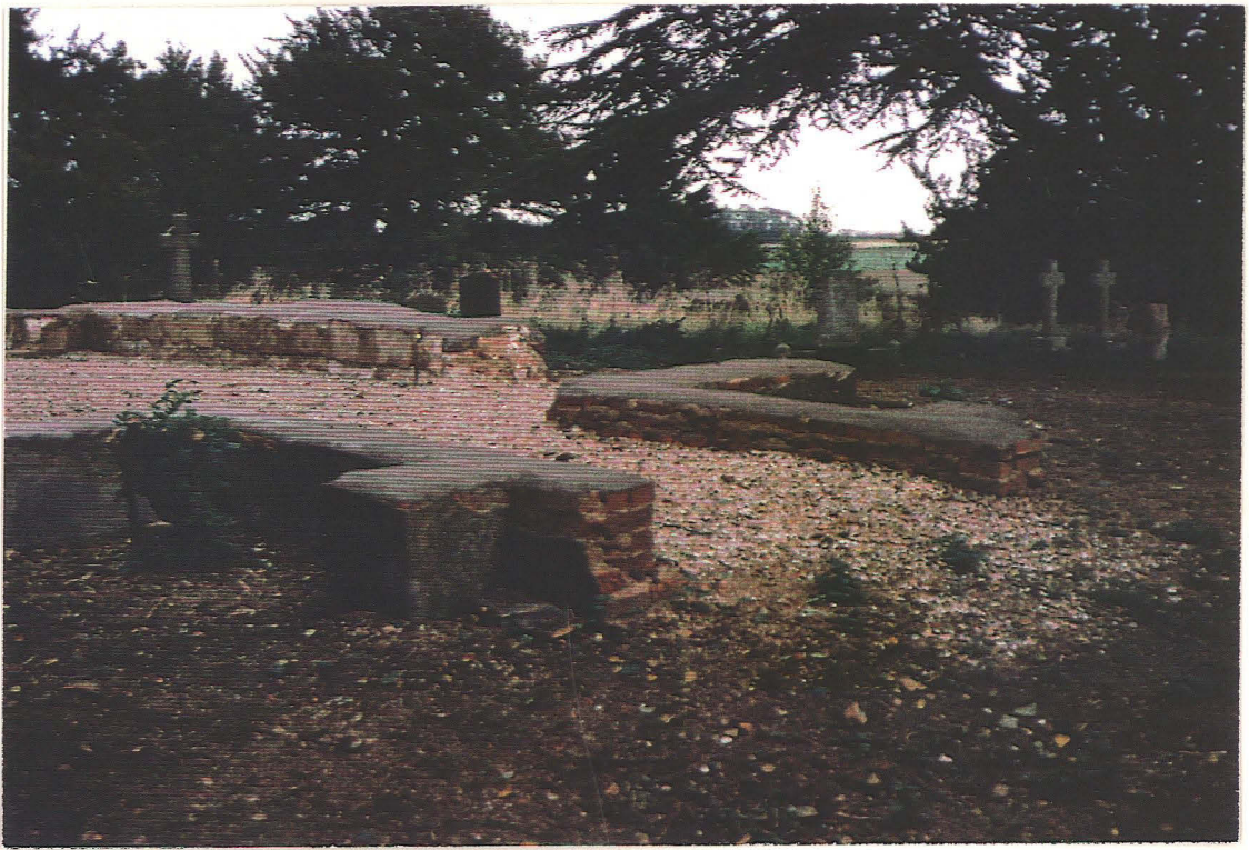
Pl. 38. Tower and nave after landscaping.
