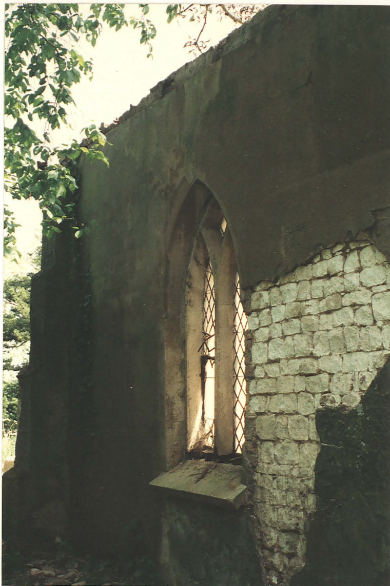
Pl.16. Nave north wall (exterior), east window, brick surround.
