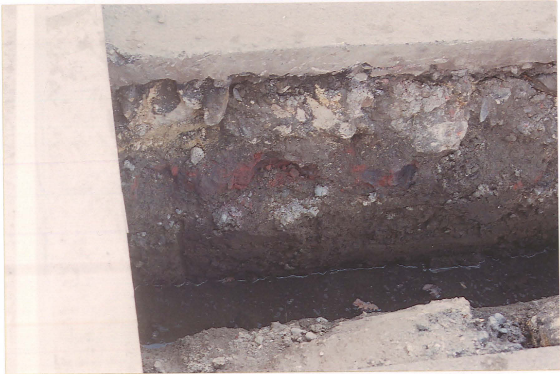
Pl. 15 Brick rubble over a thin band of gravel at (24), 50m north of the junction with Newark Road.
