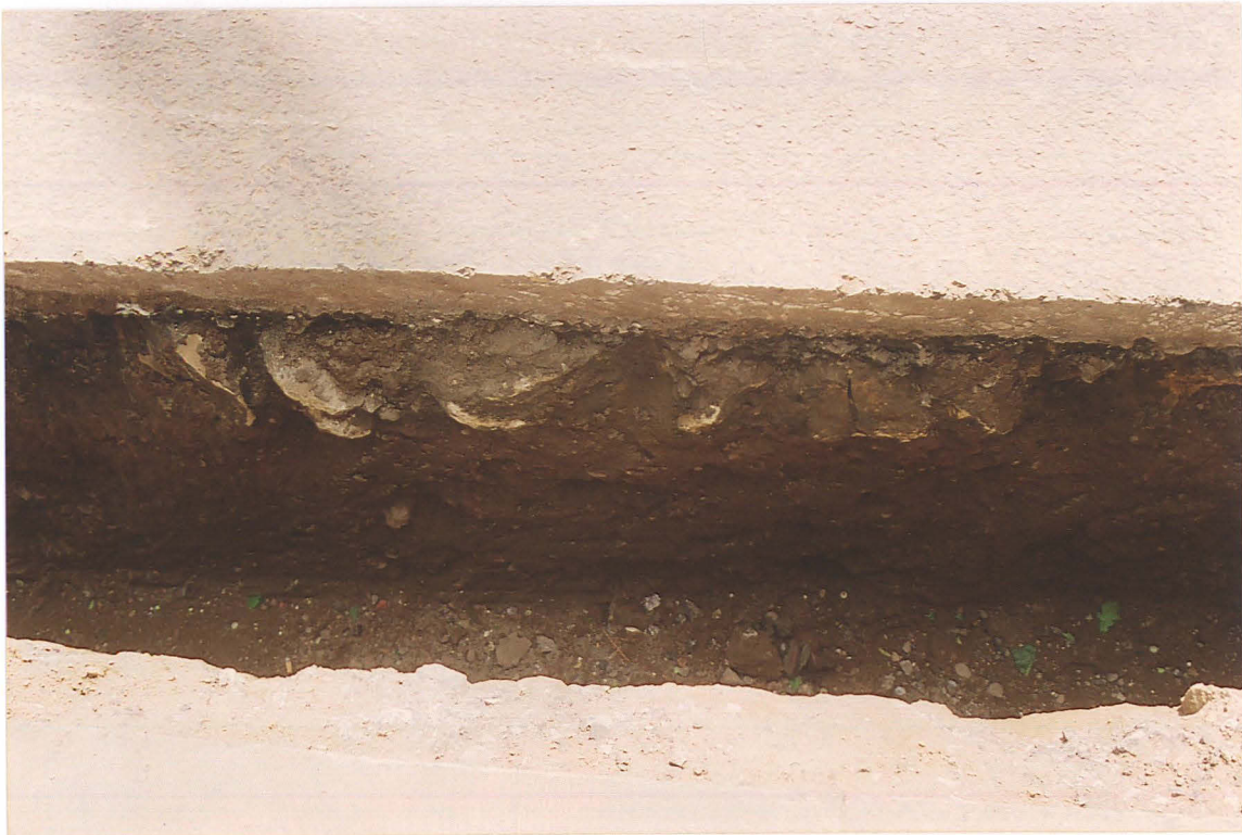
Pl. 12 South of 6 Doddington Road (16), the rubble bedding for the road lay on loamy sand.
