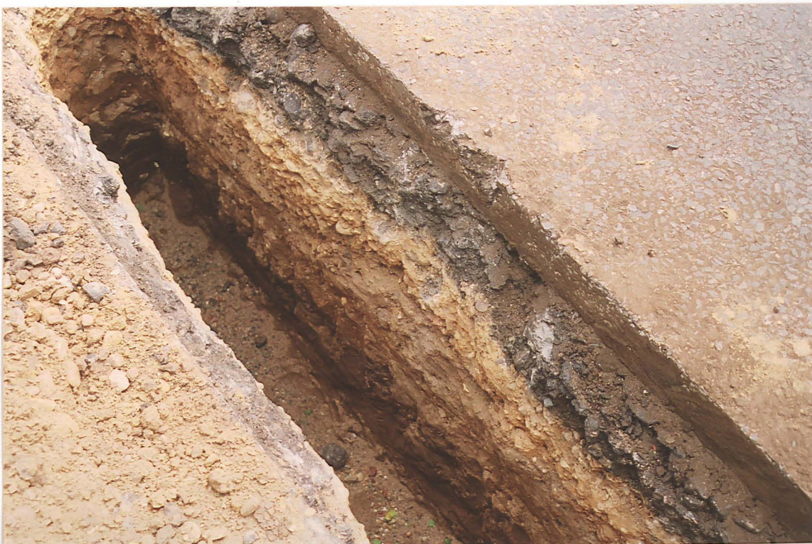
Pl. 6 Near the Waggon and Horses (5), the modern road lies on a thin layer of gravel, with brown loam below.
