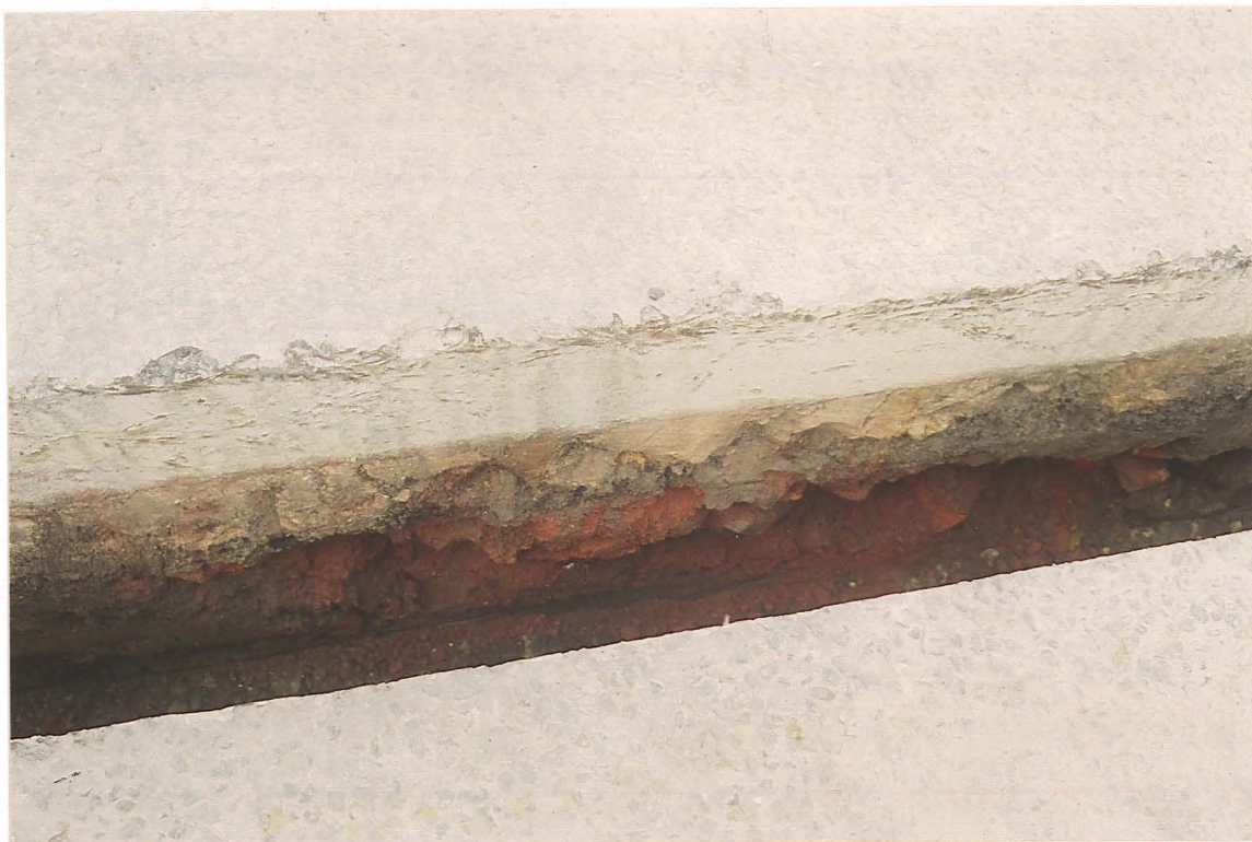
Pl. 4 Burnt material at (3), between the clinker and the underlying dark silt.
