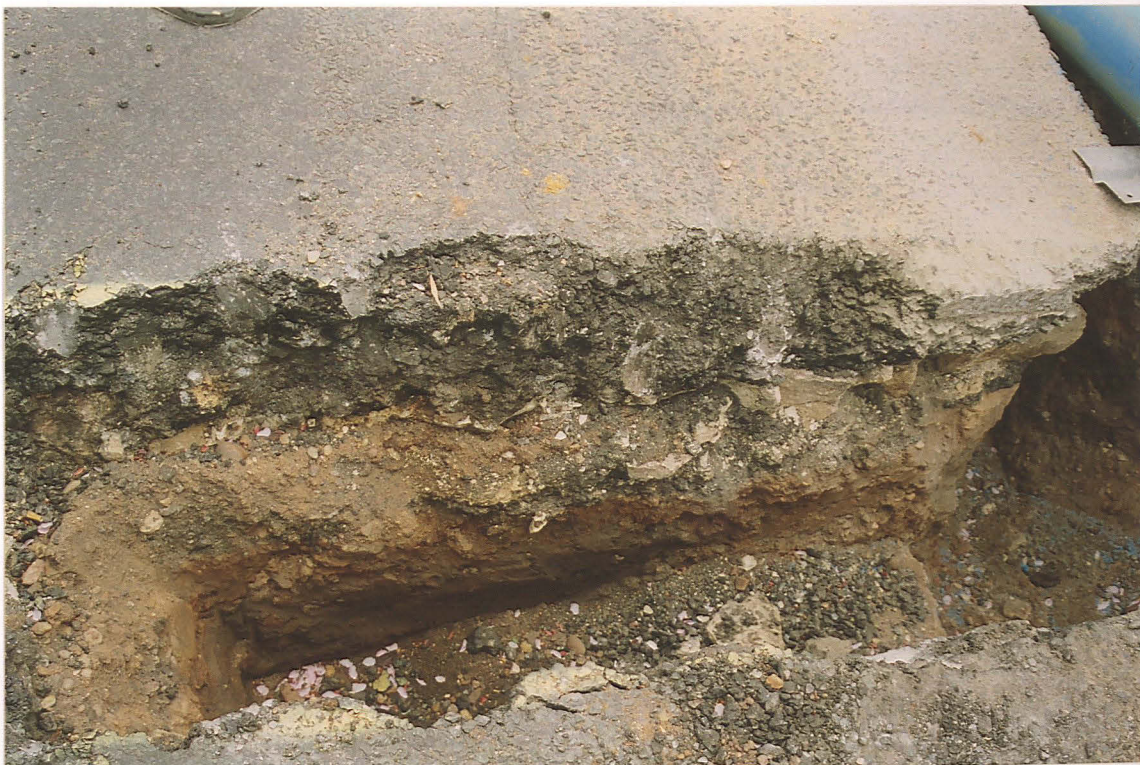
PI. 10 Mixed gravel was recorded in the trench face near 406 Newark Road (14).
