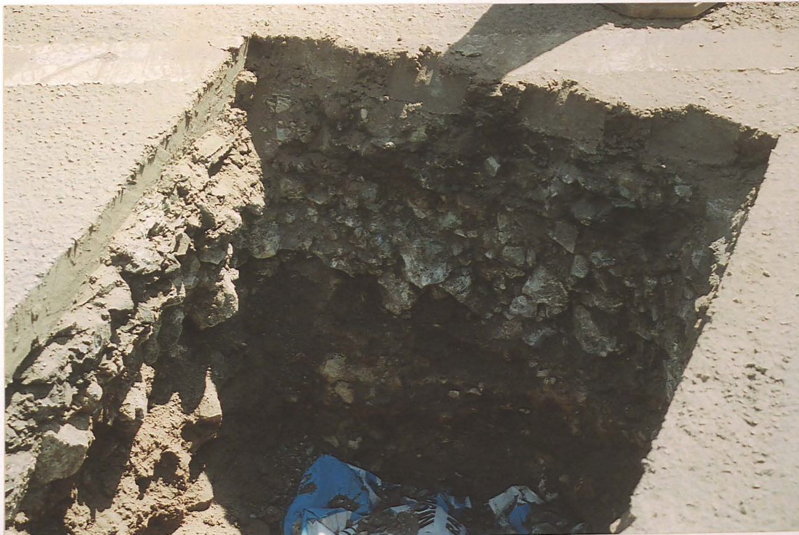
PI. 2 Compact layers of soil, gravel and stone chips below the centre of the modern road and its limestone rubble bedding layer, at Eastgate (1), looking south.
