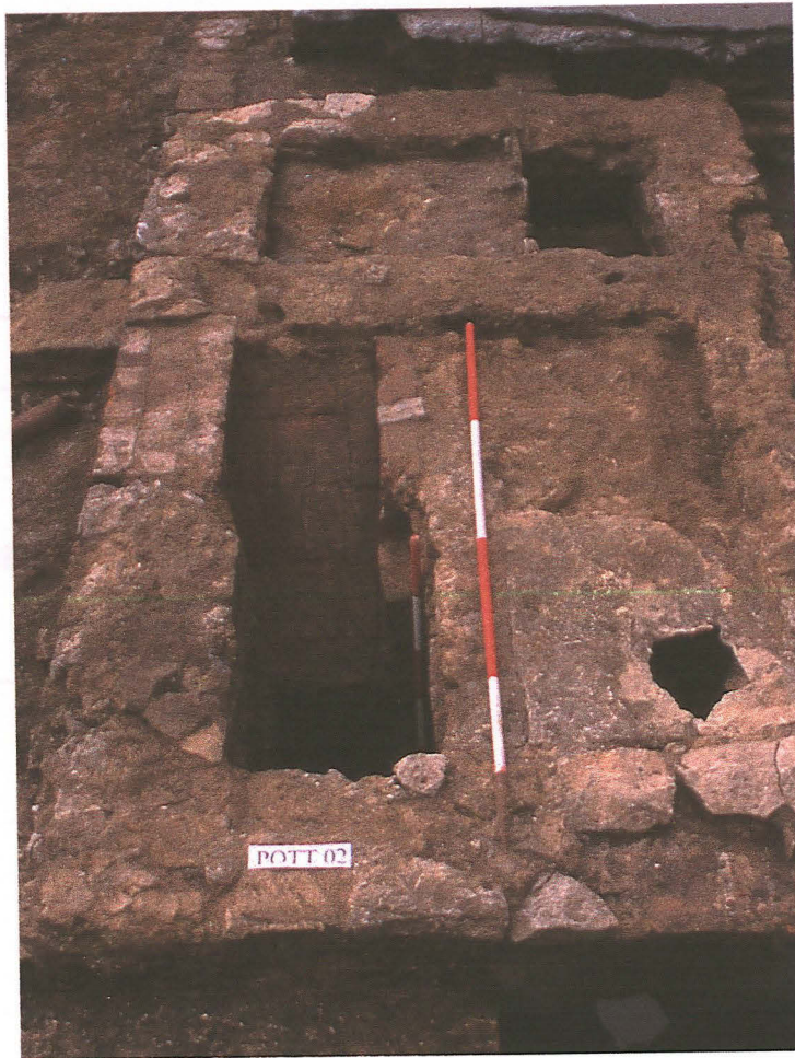
Plate 3: Toilet block (1000), looking into the septic tank from the boys' end of the structure, looking south.
