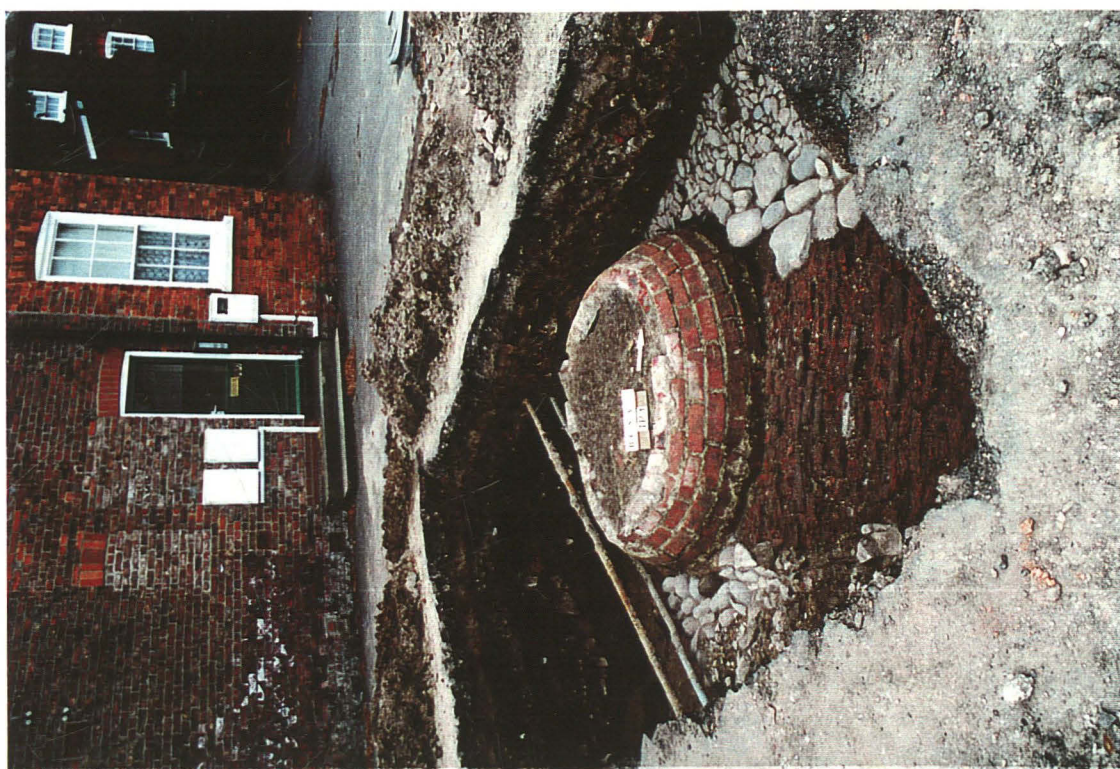
Plate 1: General view of evaluation Trench 1 following excavation, with soft water cistern (1019) at centre, truncating brick path (1016) and cobbled surface (1014)/(1015). The green door in the background is the rear entrance to the headmaster's former residence constructed in 1829, looking west.
