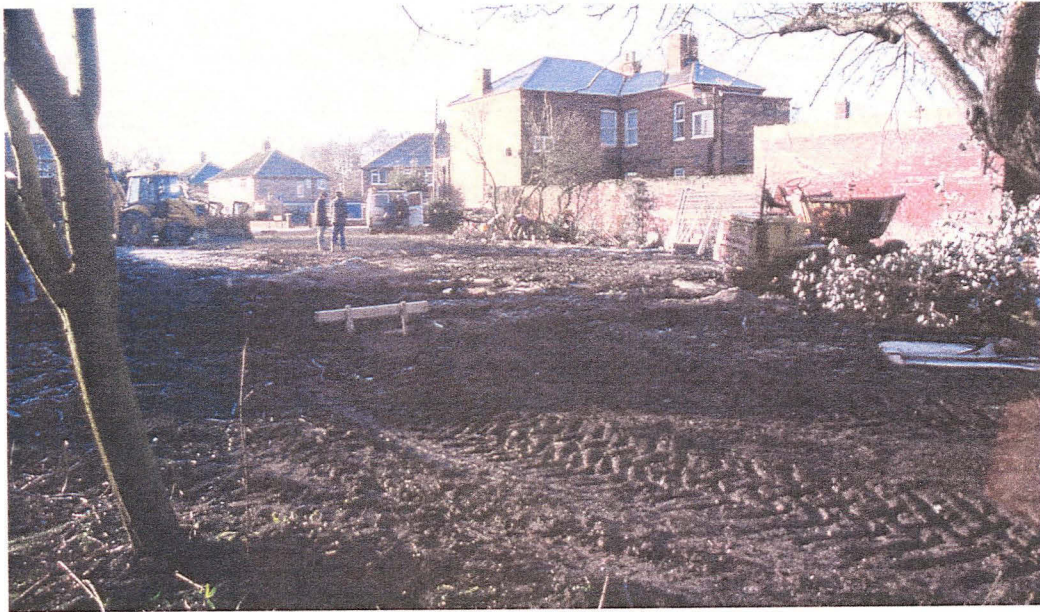
Plate 1 General view of site prior to groundworks
