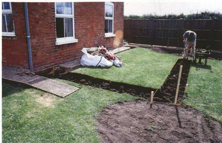
Plate 1 - General view of the development, looking northeast
