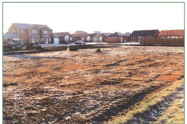
Pl. 4: Stripped area, Plots D34-D37, looking west-south-west
