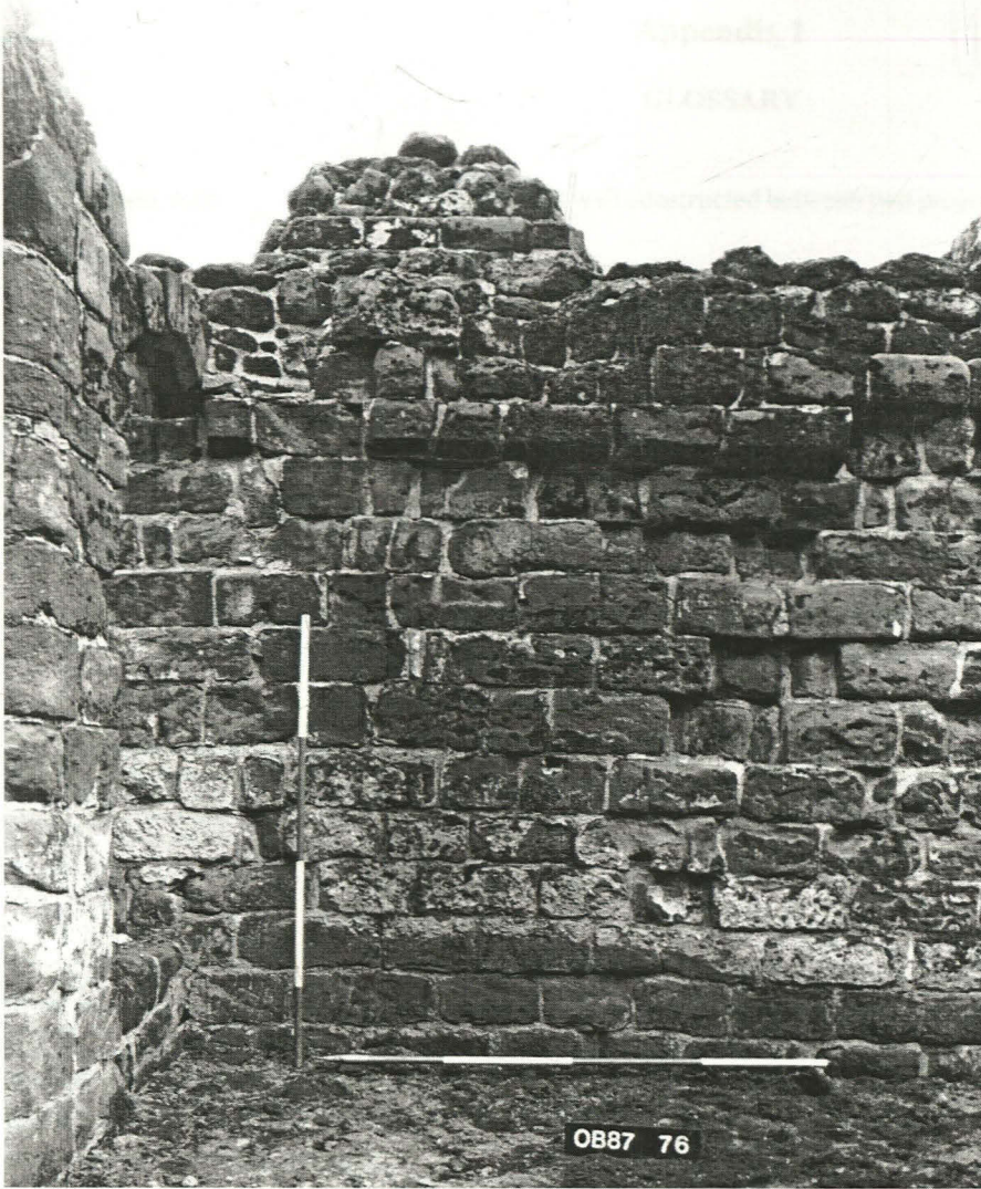
Plate 3 Interior of South Tower, east wall, showing window reveal and extant arch on left. Looking east. [Photo: English Heritage]
