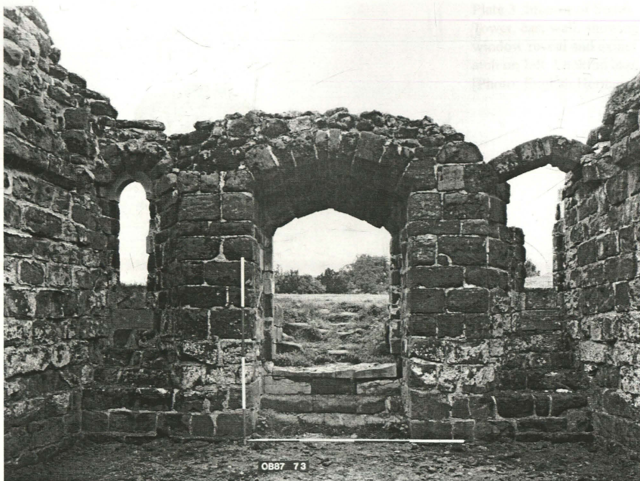
Plate 1 Interior of South Tower, showing extant window arch on right. Looking north. [Photo: English Heritage]
