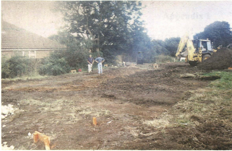
Plate 1 - General view of the development area, looking northwest
