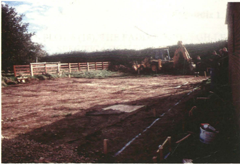
Plate 1 - General view of the development area, looking north-east
