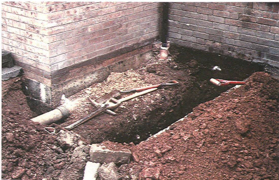
Plate 2 General view of footing for meter housing, looking south.
