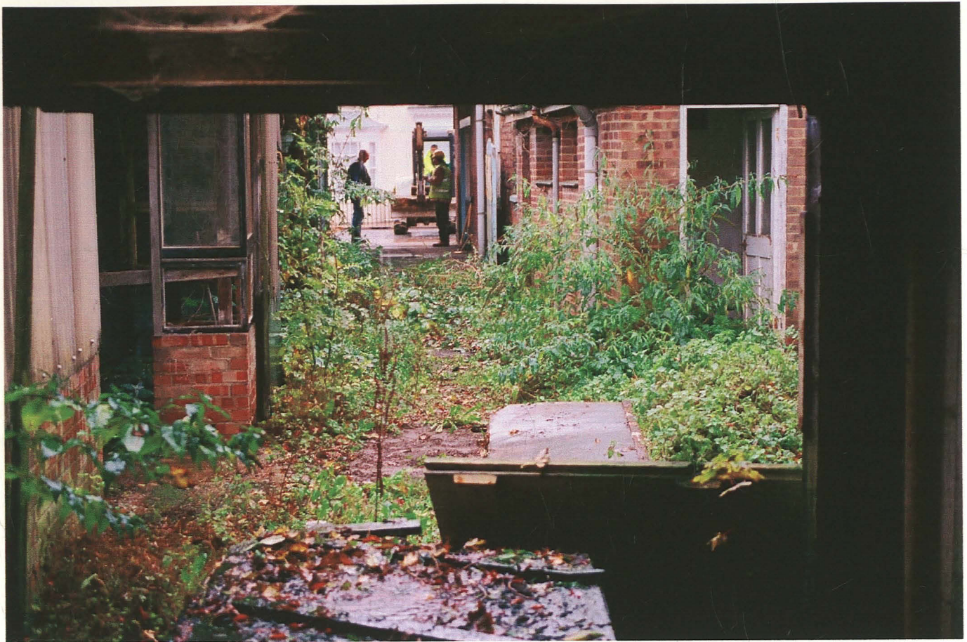
Pl. 2 General view along alley between Nos 11 and 13 Market Street, looking south.
