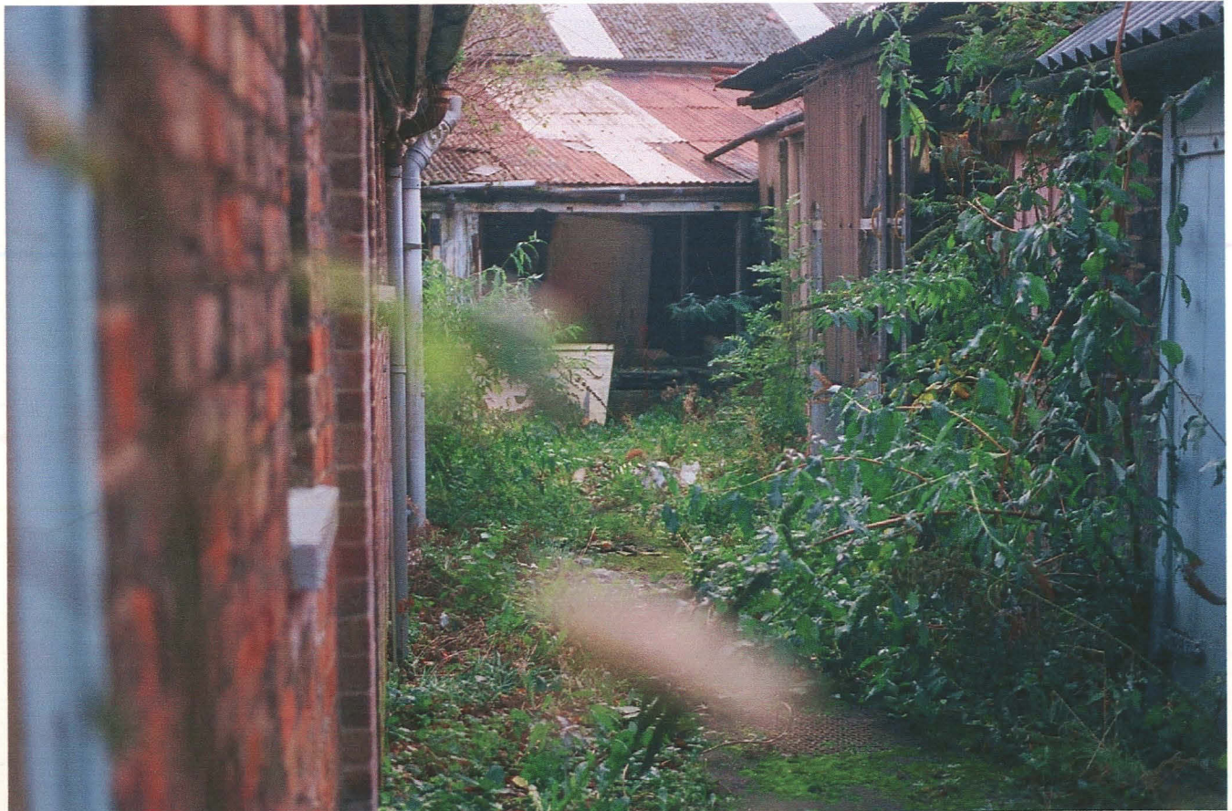
Pl. 3 General view of yard at rear of 11-13 Market Street, looking south.
