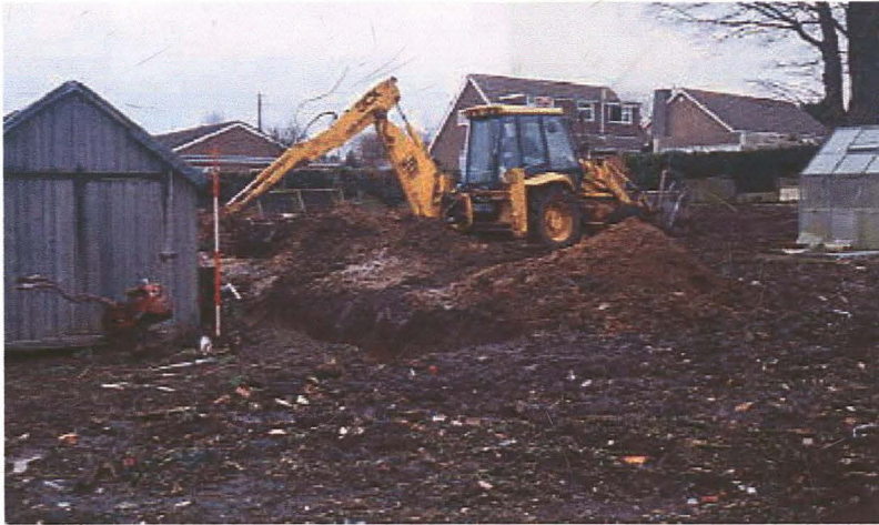
Plate 1: General shot of site with JCB at work, looking NE.
