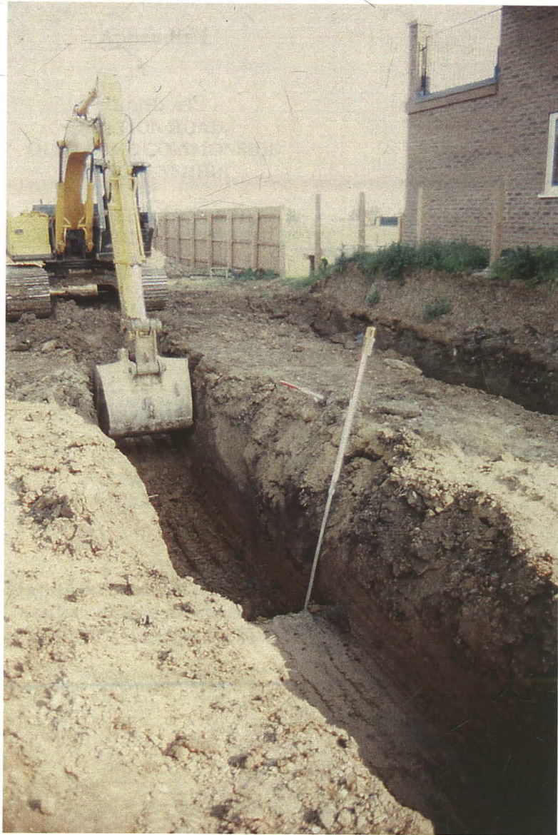
Plate 1 General view of dyke (005) during groundworks looking northeast
