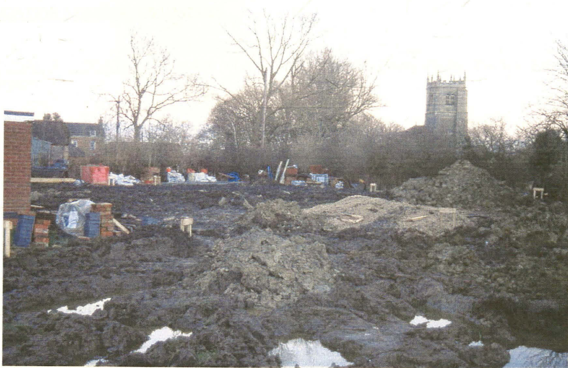
Plate 1 General view of development, looking east.
