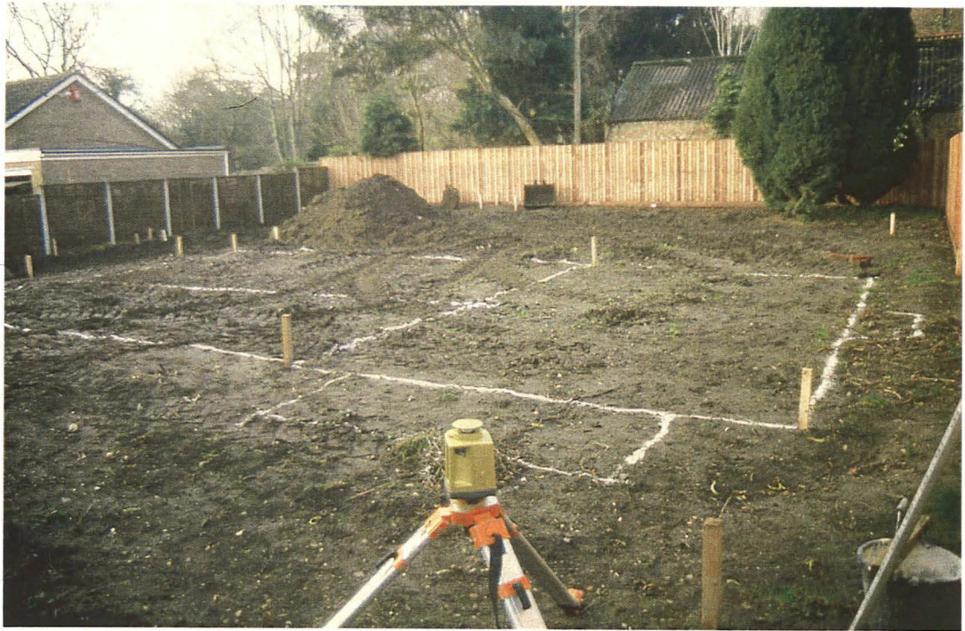
Plate 1 West facing view across site prior to groundworks
