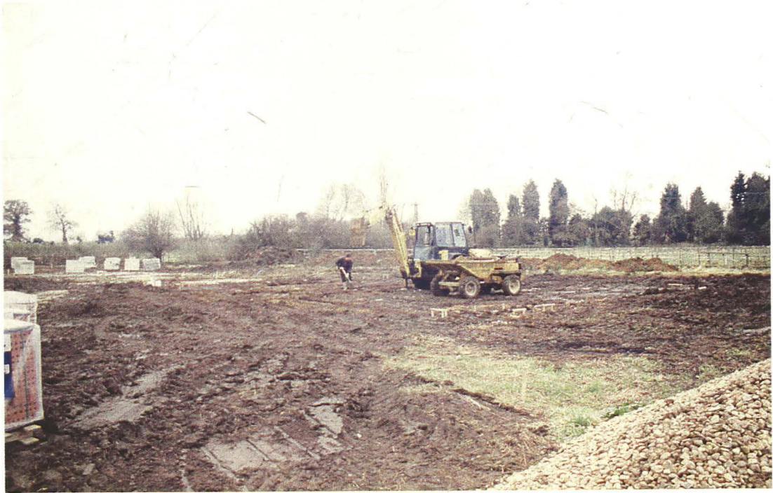
Plate 1 General View Plot 4 prior to excavation, looking southwest
