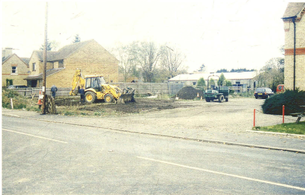
Plate 1 General view of the development, looking northeast
