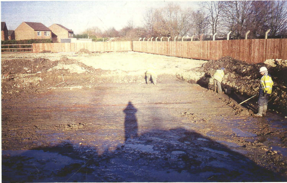
Plate 4 Working shot of Area 3 showing Structure 1 during cleaning, looking north.
