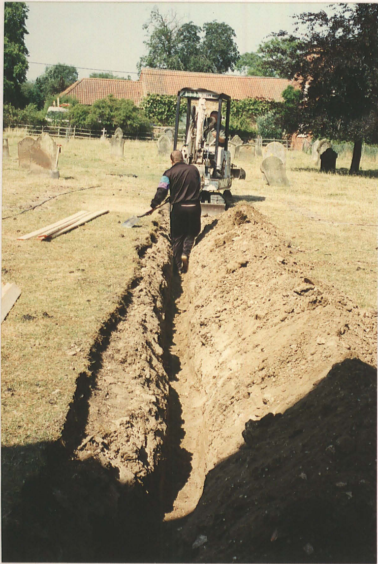
Pl. 5 Excavation of the cable trench across the former nave area
