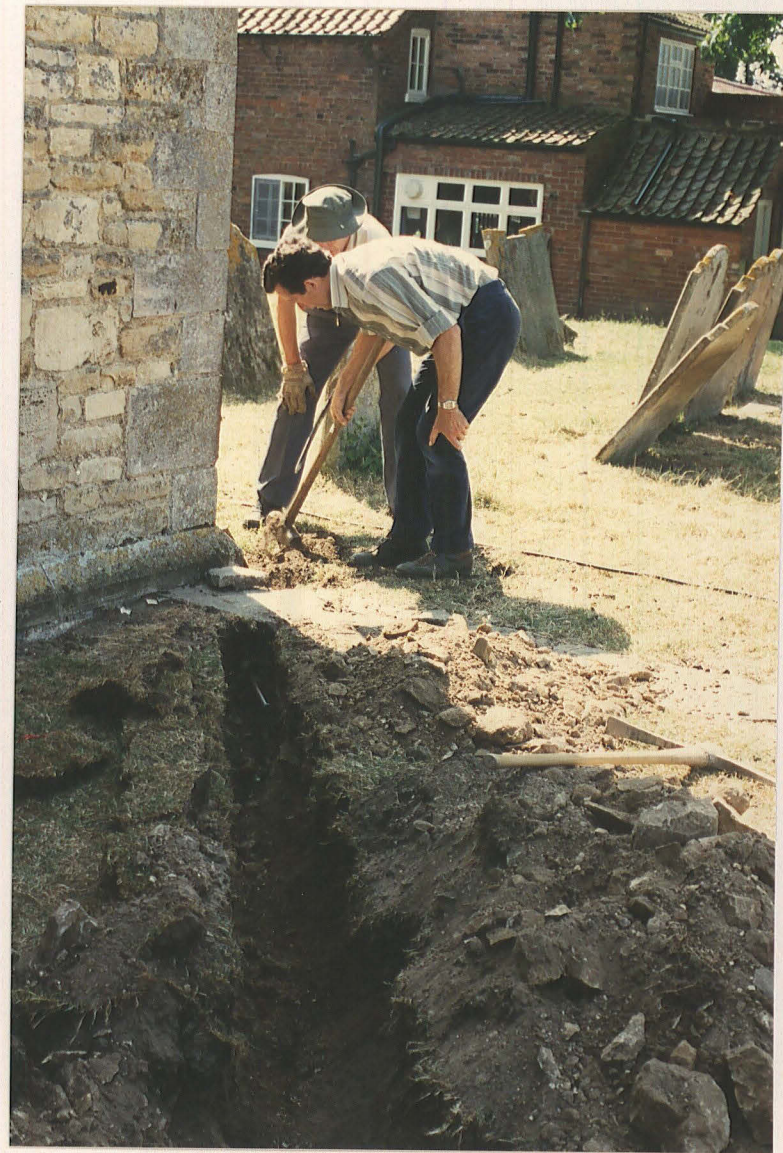
Pl. 5 Excavation of the cable trench across the former nave area
