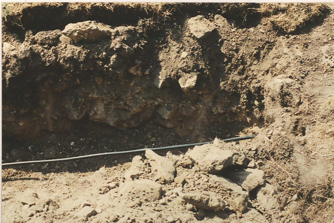
Pl. 10 Stone rubble and mortar beside west wall of demolished nave (looking south)
