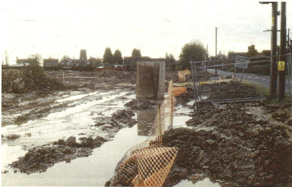
Plate 1 General view of development at commencement of groundworks, looking southwest
