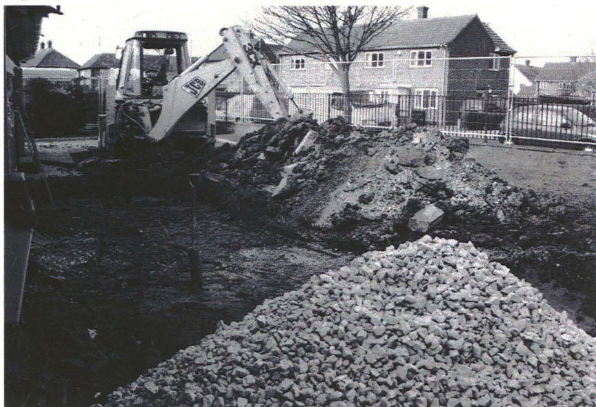
Pl. 1 : General shot of site during excavation of footings. Looking south.
