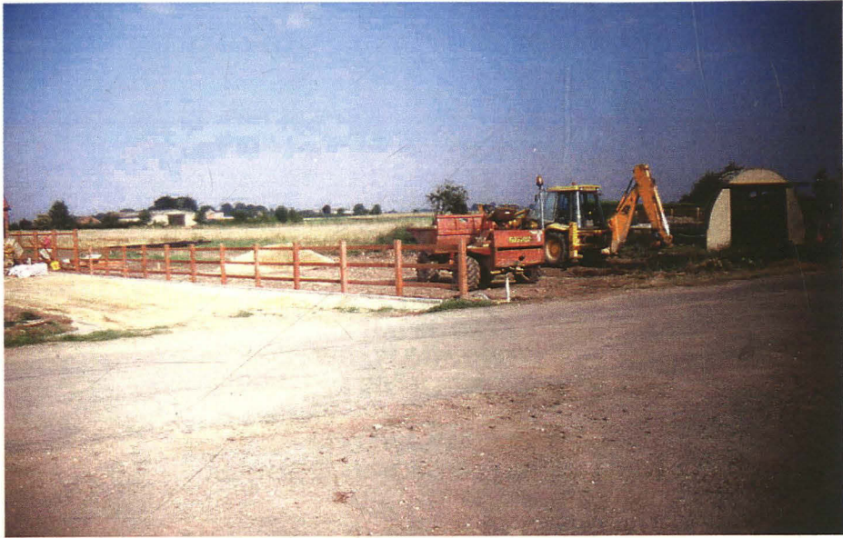
Plate 1 General view excavation area looking southwest
