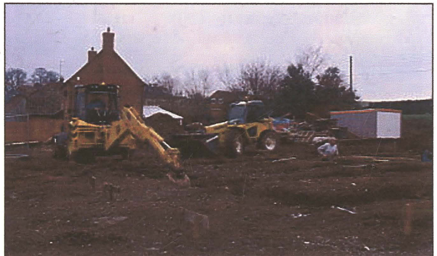
Plate 2 (right): General view of the houseplot during excavation, looking SSW.
