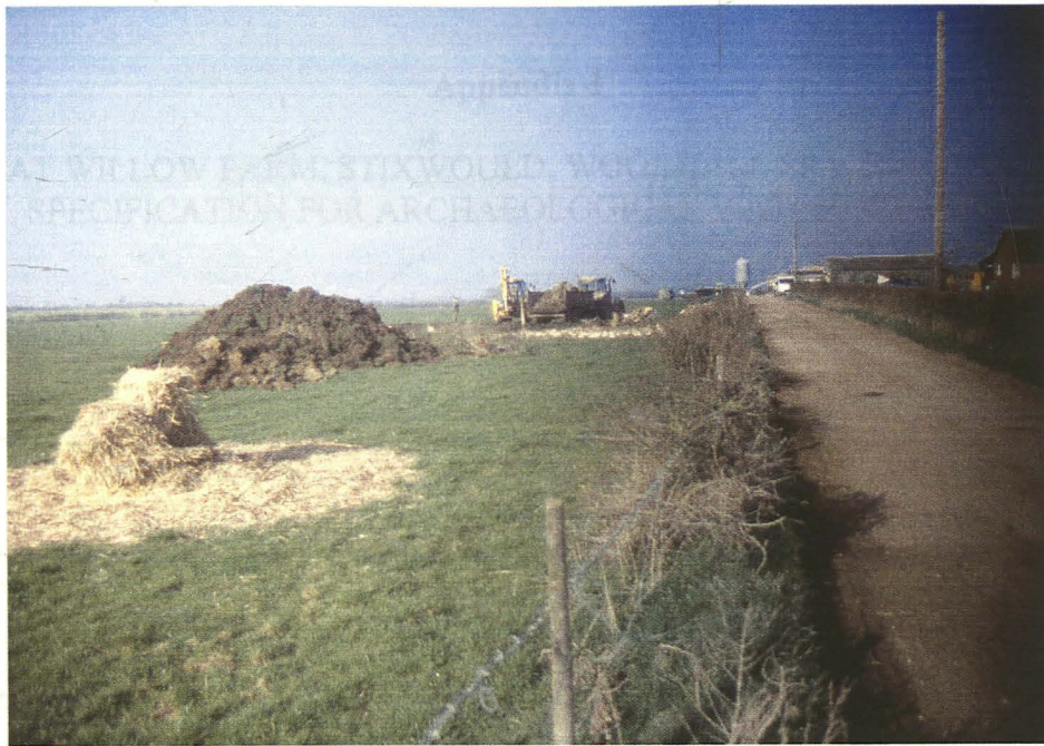
Plate 1 - General view of the development, looking northwest
