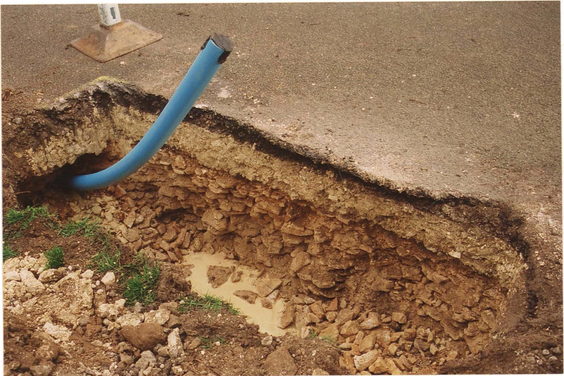
Pl. 4 Dense limestone brash in the southern face of Trench 3.
