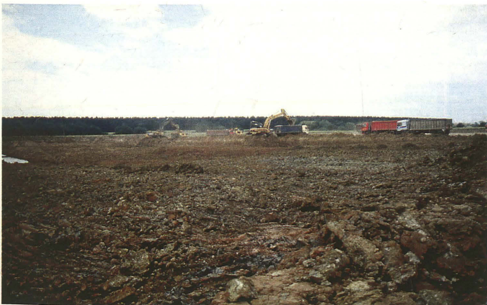
Plate 3 General view of topsoil stripped area
