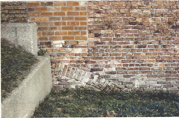
Plate 11 - View of the infilled western arch for access to the water wheel, looking north
