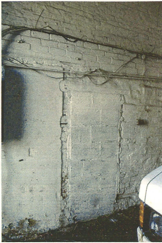
Plate 8 - Interior view showing the blocked door on the eastern wall
