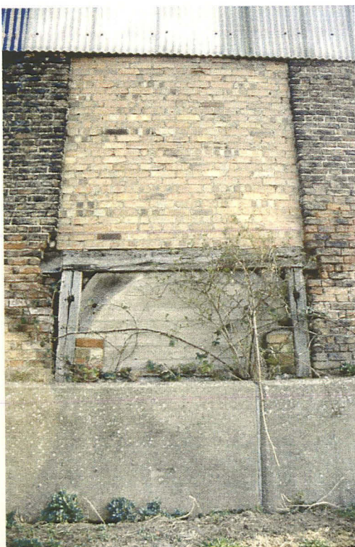
Plate 13 - Detail of blocked doorway, looking east
