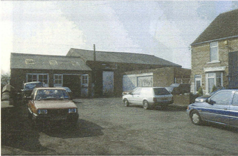
Plate 5 - The mill and associated buildings showing the principal entrance, looking southwest
