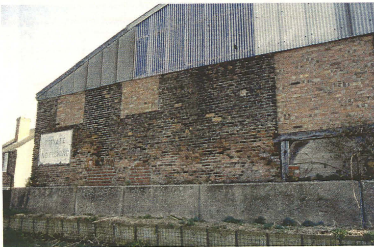
Plate 12 - The west elevation, looking northeast
