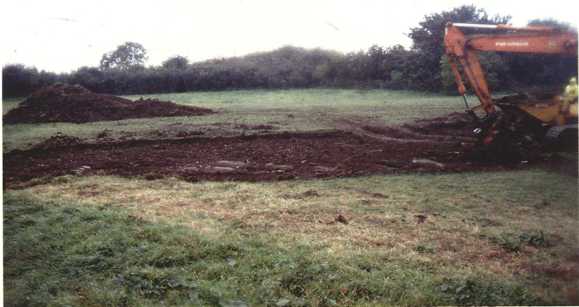
Plate 2 General view of stripping in progress
