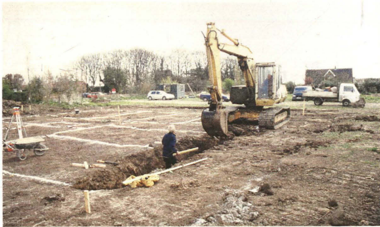
Plate 1 General view of site on commencement of excavation looking southeast
