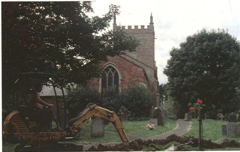
Plate 1 - Excavation of the cable trench , looking southwest towards St. Peter's church
